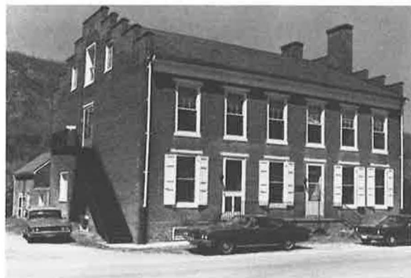
Wilson Warehouse, Buchanan, Botetourt County
