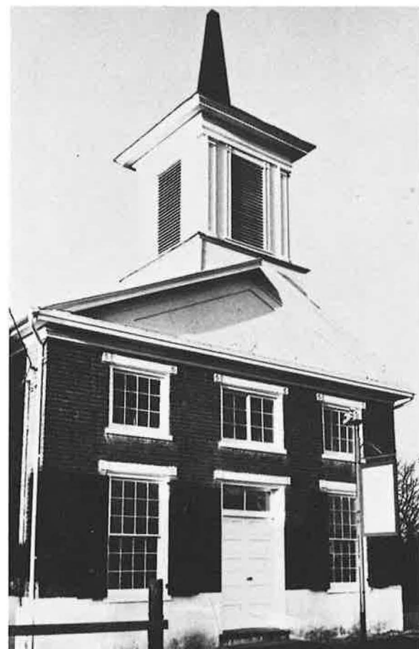
Bedford Historic Meeting House, Bedford
