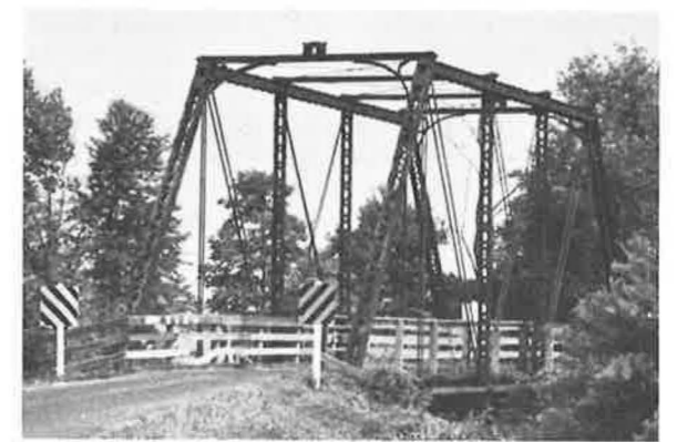
Goshen Land Company Bridge, Rockbridge County
