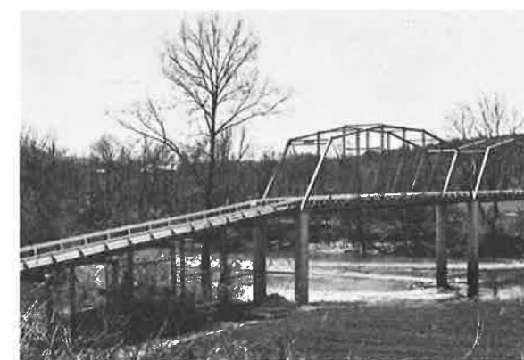
Mansion Truss Bridge, Campbell County
