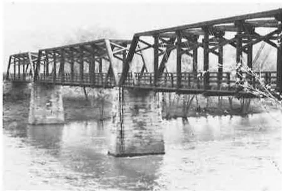
Springwood Truss Bridge, Botetourt County
