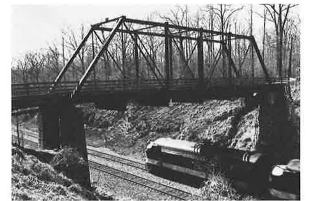
Oak Ridge Railroad Overpass, Nelson County
