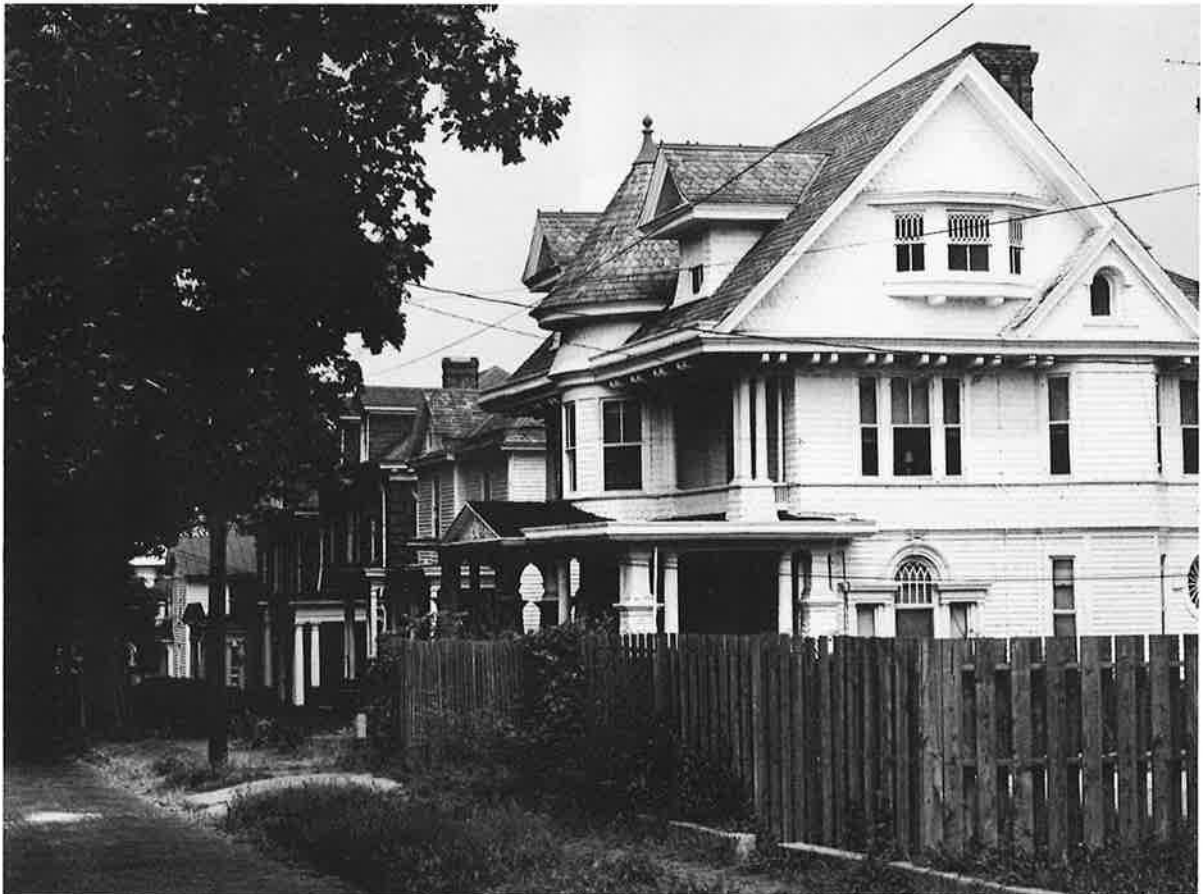
Clay Street, Diamond Hill Historic District, Lynchburg
