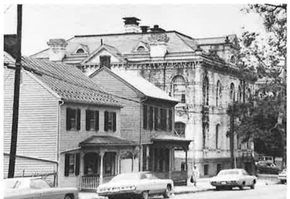
203-213 S. Cameron St., Winchester Historic District
