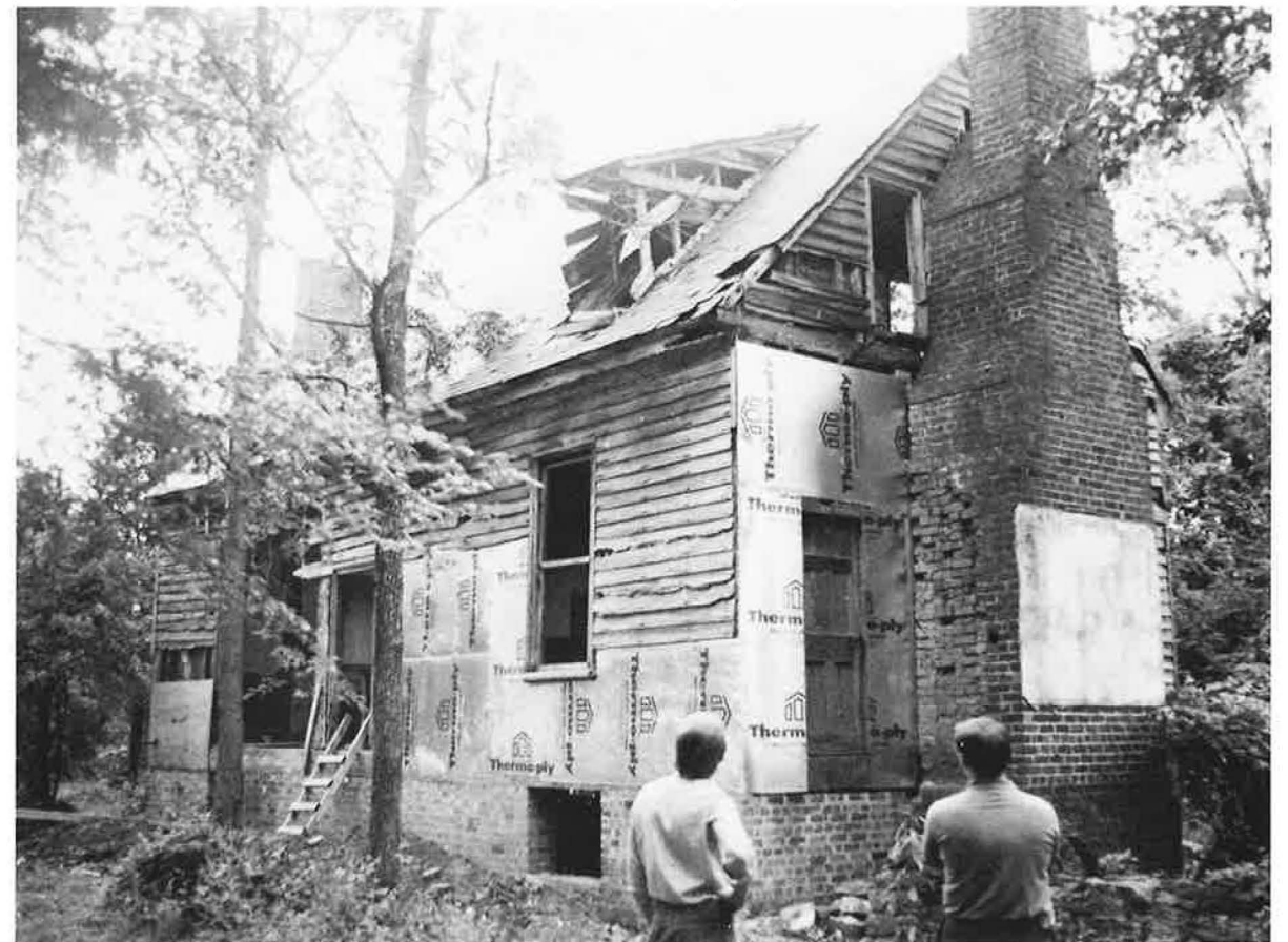
Restoration underway on the Peter Francisco House, Buckingham County
