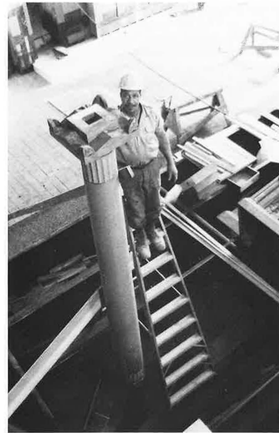
Restoring the Gallery of Monumental Church, Richmond
