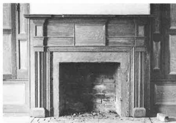
Oak Hill, second-floor bedroom fireplace
