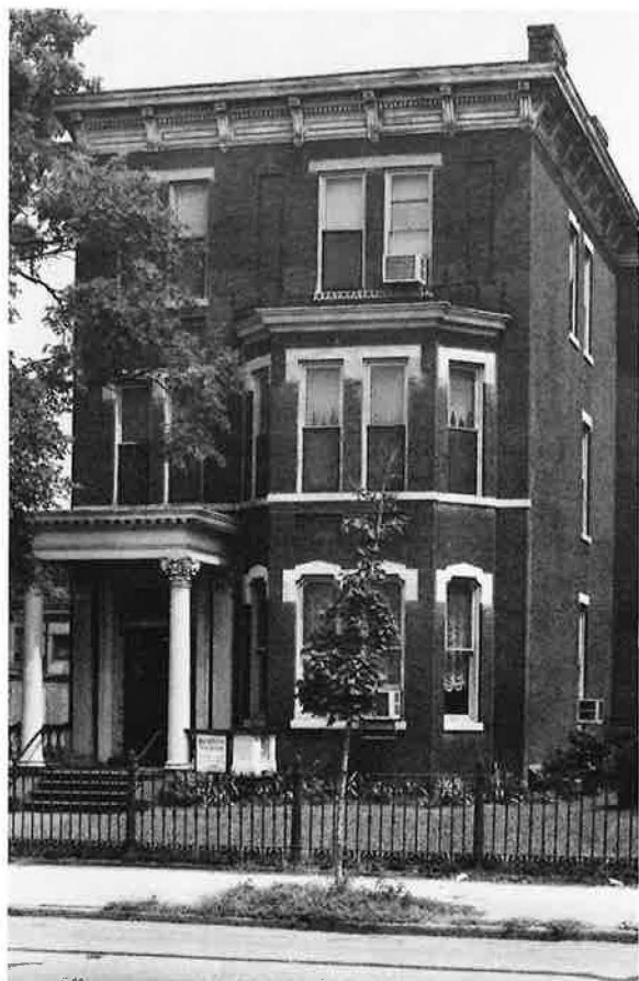
Morton's Tea Room, 0-100 Block East Franklin Street Historic District, Richmond
