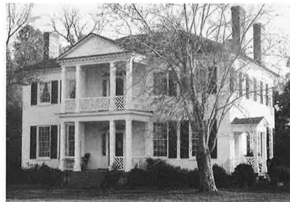
Magnolia Grange, Chesterfield County
