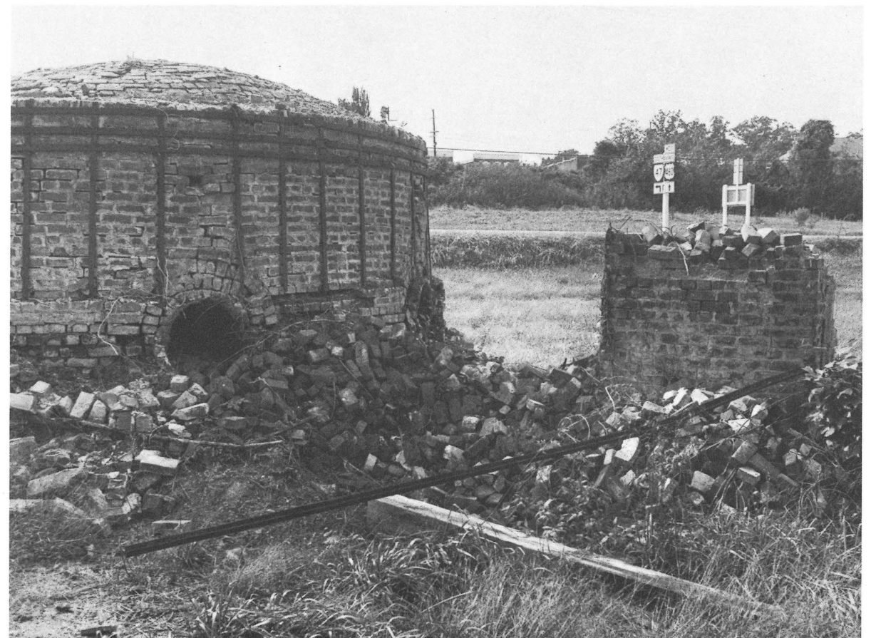
Kiln and chimney, Pamplin Pipe Factory, Appomattox County
