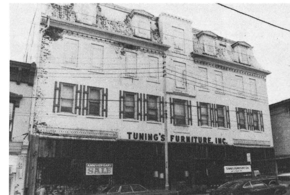
Eakleton Hotel, Staunton, before rehabilitation
