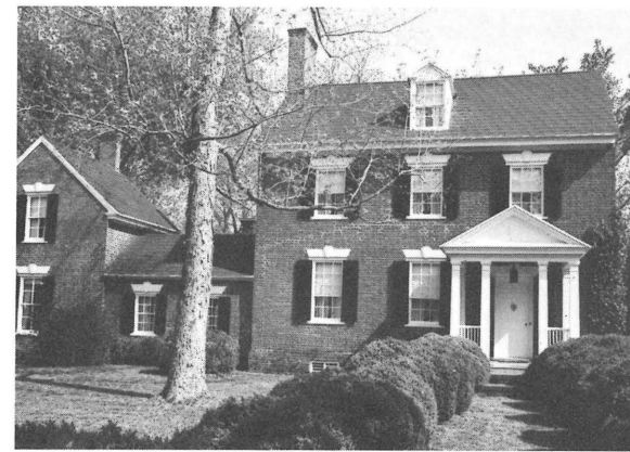
Drummond House, Accomac Historic District
