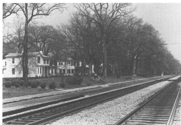
West Side of South Center Street, Looking North, Ashland Historic District
