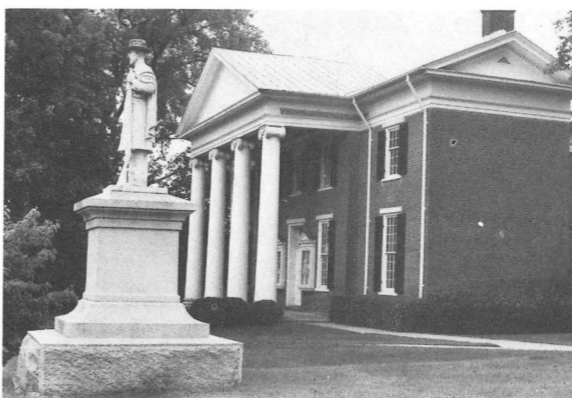
Halifax County Courthouse
