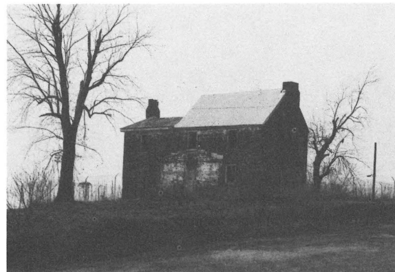
Conner House, Prince William County
