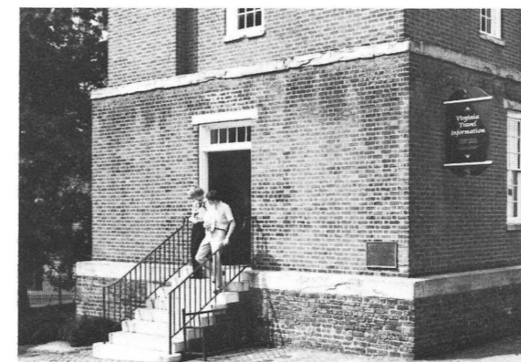
The Bell Tower now serves as the Virginia State Travel Service information center.
