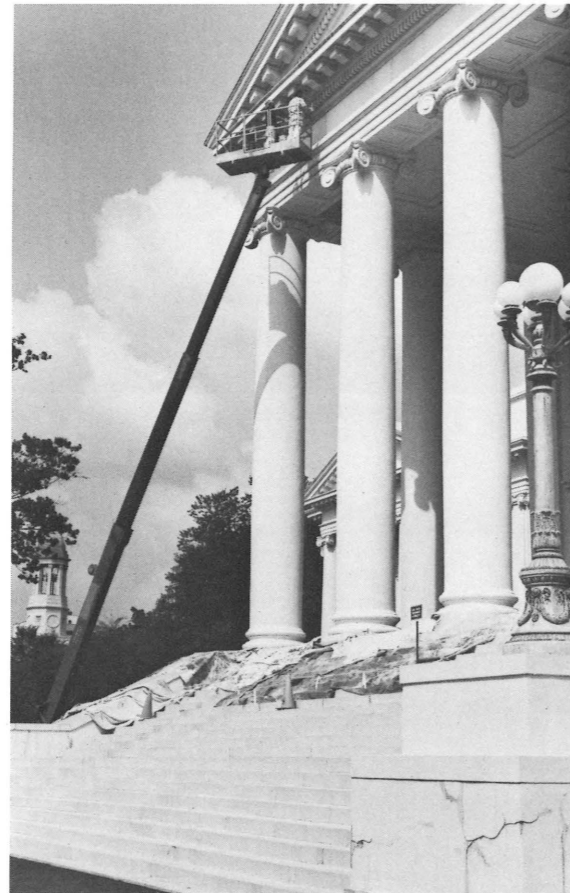
The State Capitol's stuccoed walls are being repaired and repainted.
