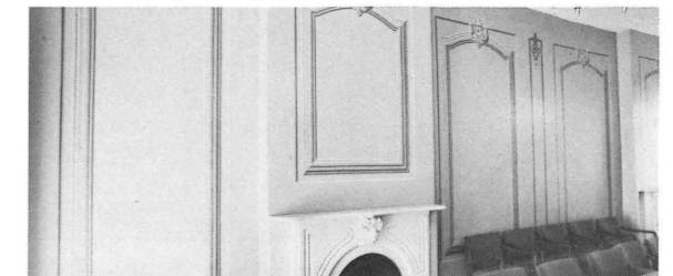
The Putney House parlor has its original trompe l'oeil panels repaired.
