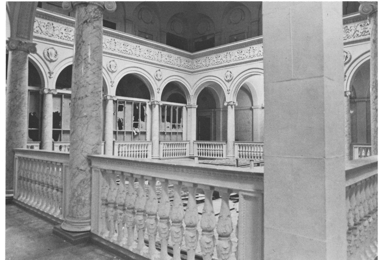
Interior view of Old City Hall, Norfolk
