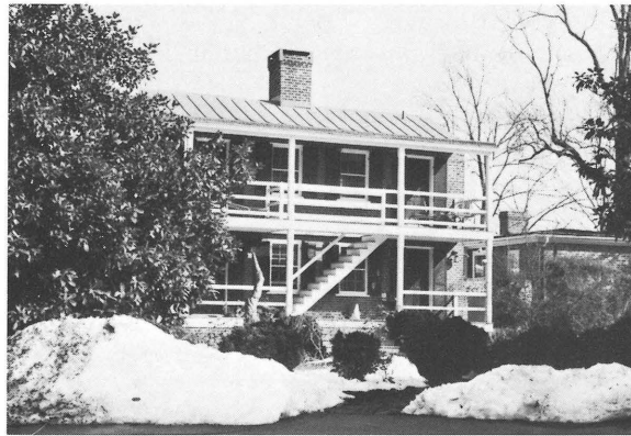
Carr's Hill Dormitory, south facade
