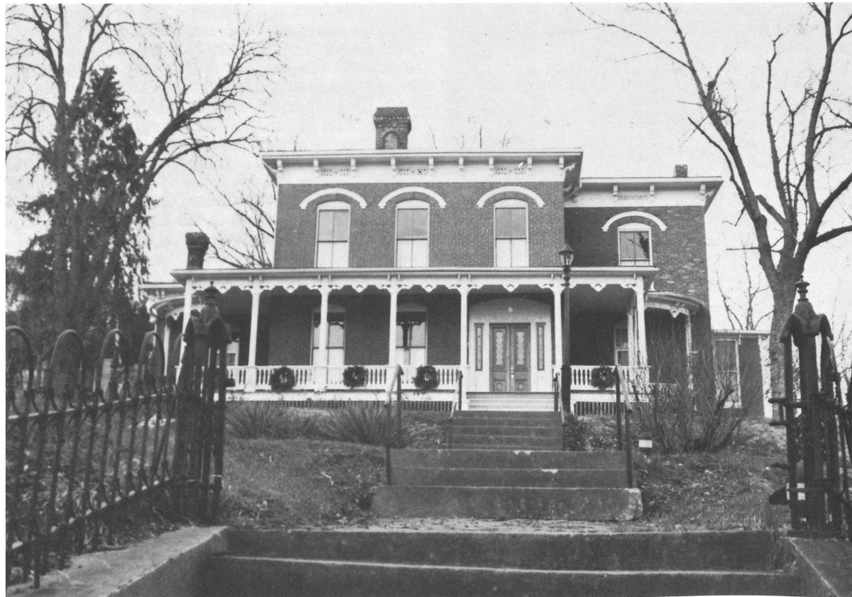
Belle Grae Inn, 515 West Frederick Street, Newtown Historic District, Staunton
