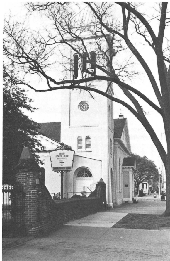
Trinity Episcopal Church on Court Street in Portsmouth. The 1830 church was listed on the Virginia and National registers in 1973.
