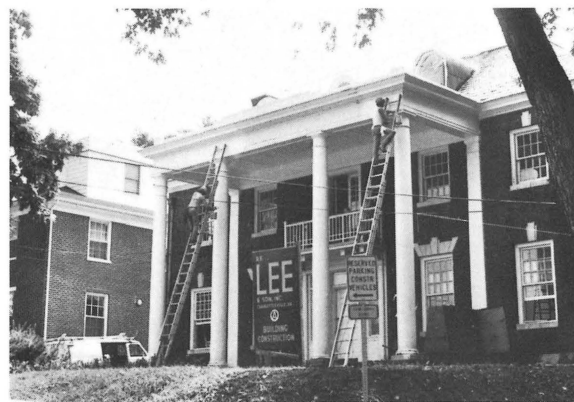
The Saint Elmo Hall, during rehabilitation, Summer 1984
