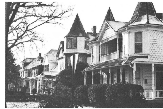
Port Norfolk Historic District was entered on the Virginia and National registers in 1983. It is the largest historic district in Portsmouth.
