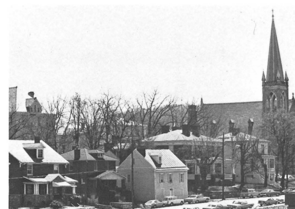
Stuart Addition, Staunton
