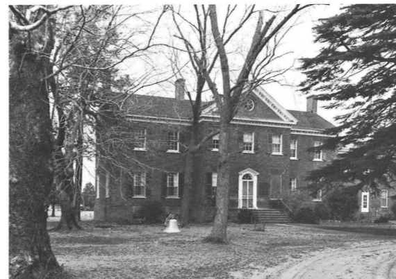
Kerr Place, Onancock, Accomack County
