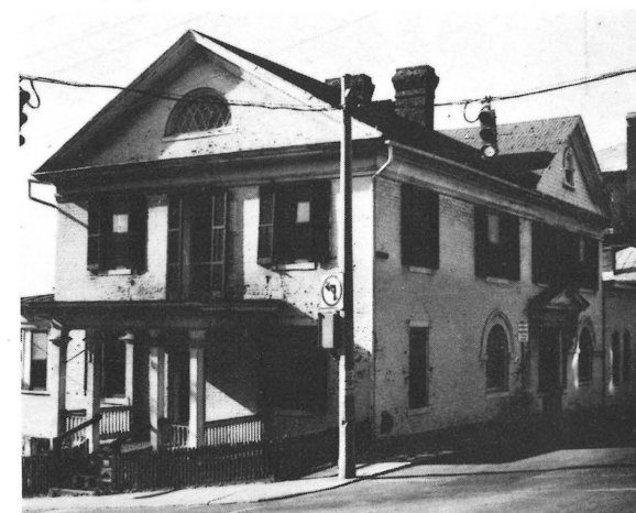
18 East Frederick Street in the Beverley Historic District in Staunton, before rehabilitation.
