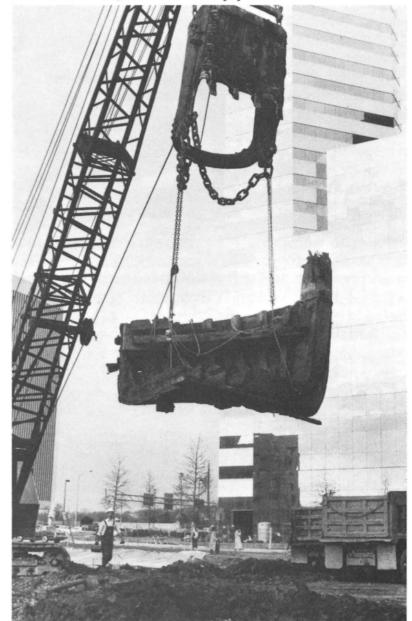
Crane lifts in tact canal boat from excavations of the James River—Kanawha Canal turning basin in downtown Richmond. Credit: Bill Lane, Richmond Newspapers
