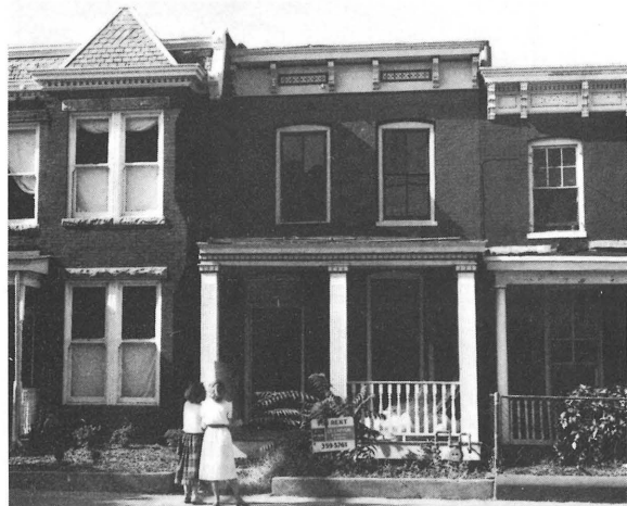
Lisa Lahendro and Dianne Pierce inspect Tax Act project at 13 1/2 West Leigh Street in Richmond's Jackson Ward.
