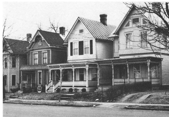
Southwest Historic District, Roanoke. View of 534-540 Mountain Avenue, looking southeast.
