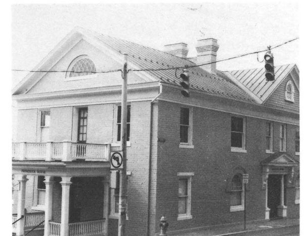
18 East Frederick Street after completion of rehabilitation project.
