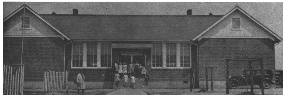
Crimora School: Fourth phase of consolidated school construction; the central auditorium that was used from 1929 to 1940 in the county. 1932 Insurance photograph.
