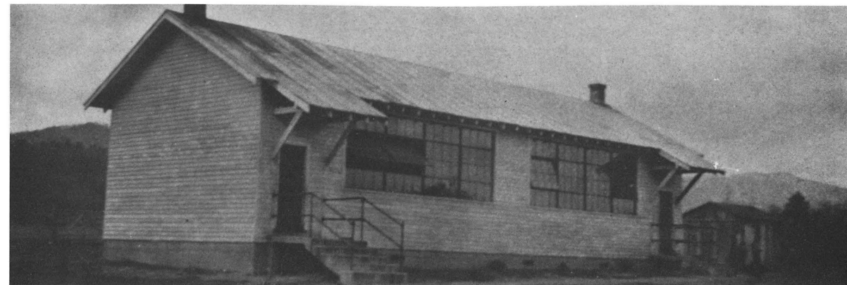
Craigsville Colored School: Two-room schoolhouse built according to guidelines and plans for the Division of School Buildings in the 1920s. 1932 Insurance Survey.
