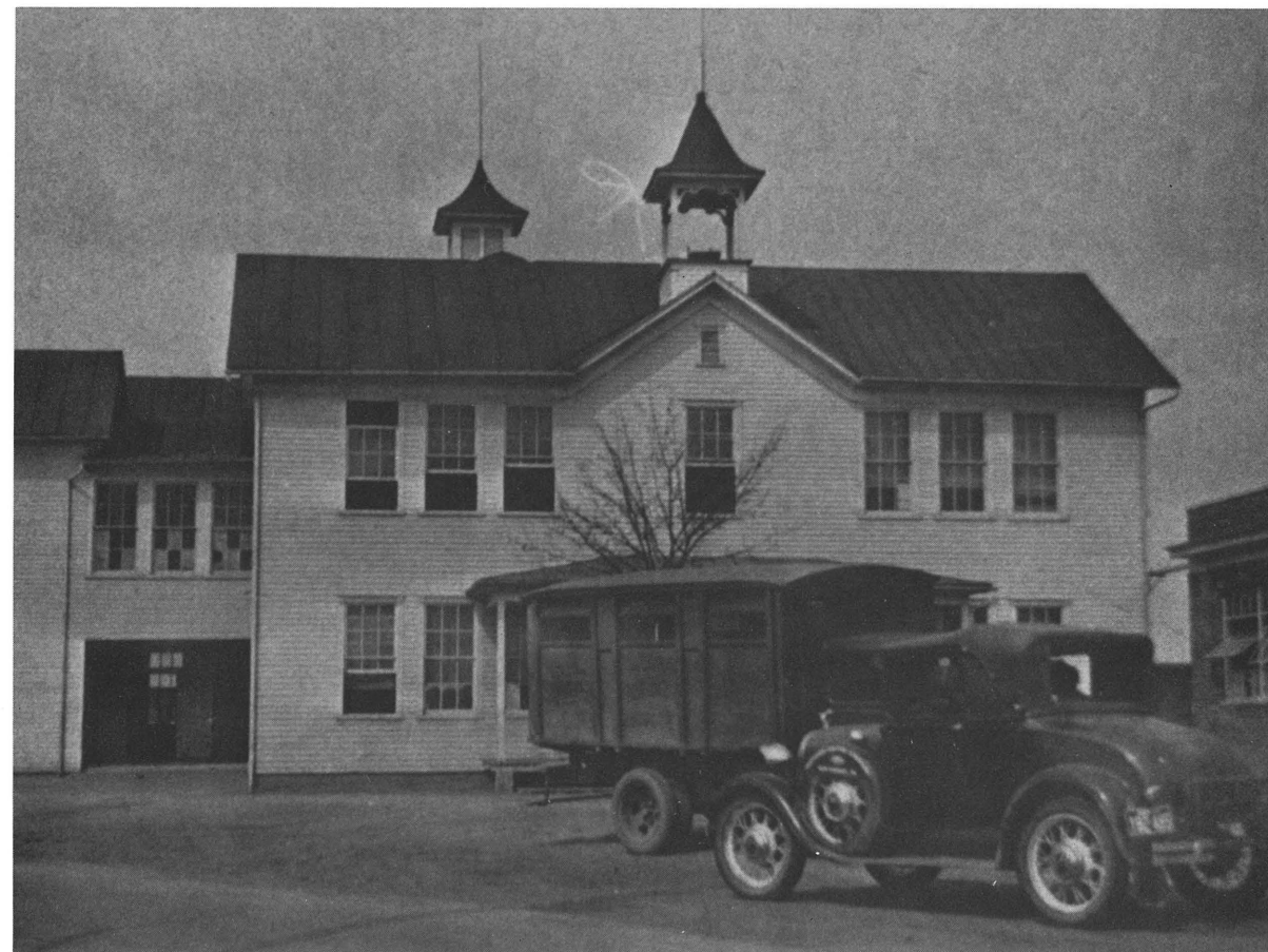
New Hope Elementary School: First stage of consolidated schools (resembling local domestic architecture). 1932 Fire Insurance Survey.
