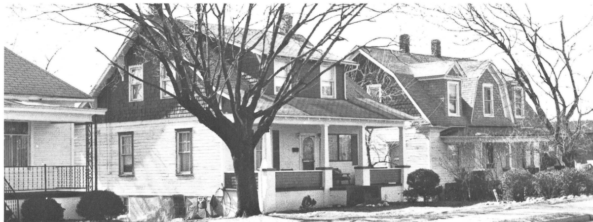
Southwest Historic District, view of 1822-26 Salem Avenue, Roanoke.
