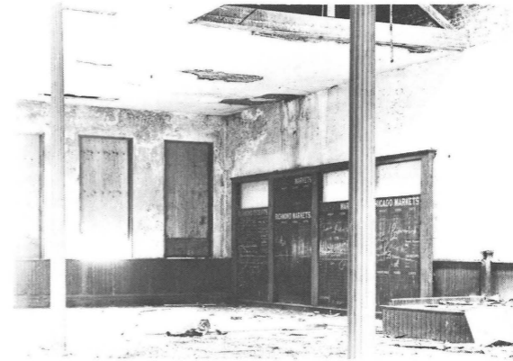
The Columbian Block, interior before rehabilitation.
