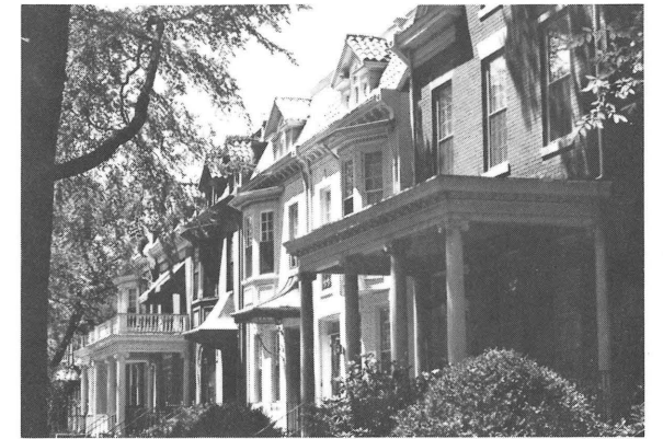
Fan Area Historic District, view of the 1800 block, Hanover Avenue.
