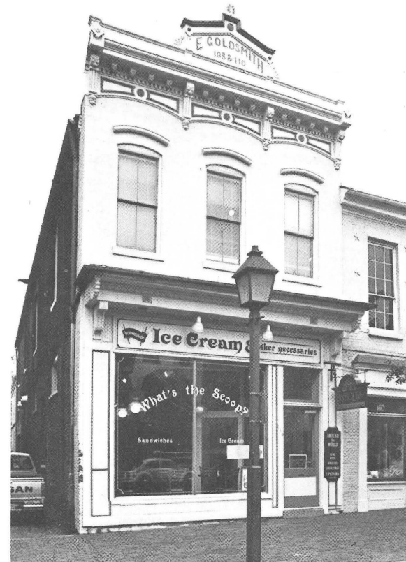
110 King Street, Alexandria, after rehabilitation. Credit: James C. Massey
