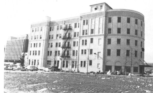
Seaboard Coastline Building, Portsmouth.
