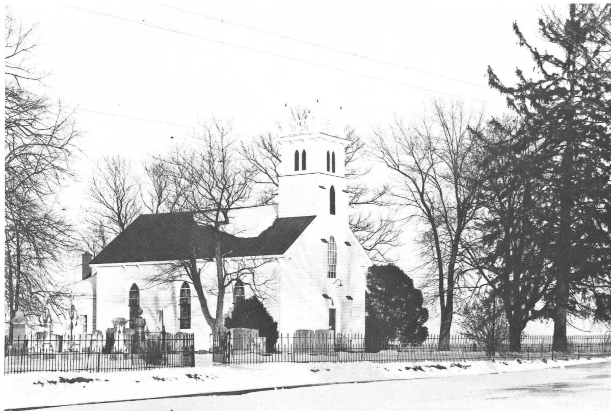
Plate Number One: Exterior of church in 1979 before restoration, showing metal siding.
