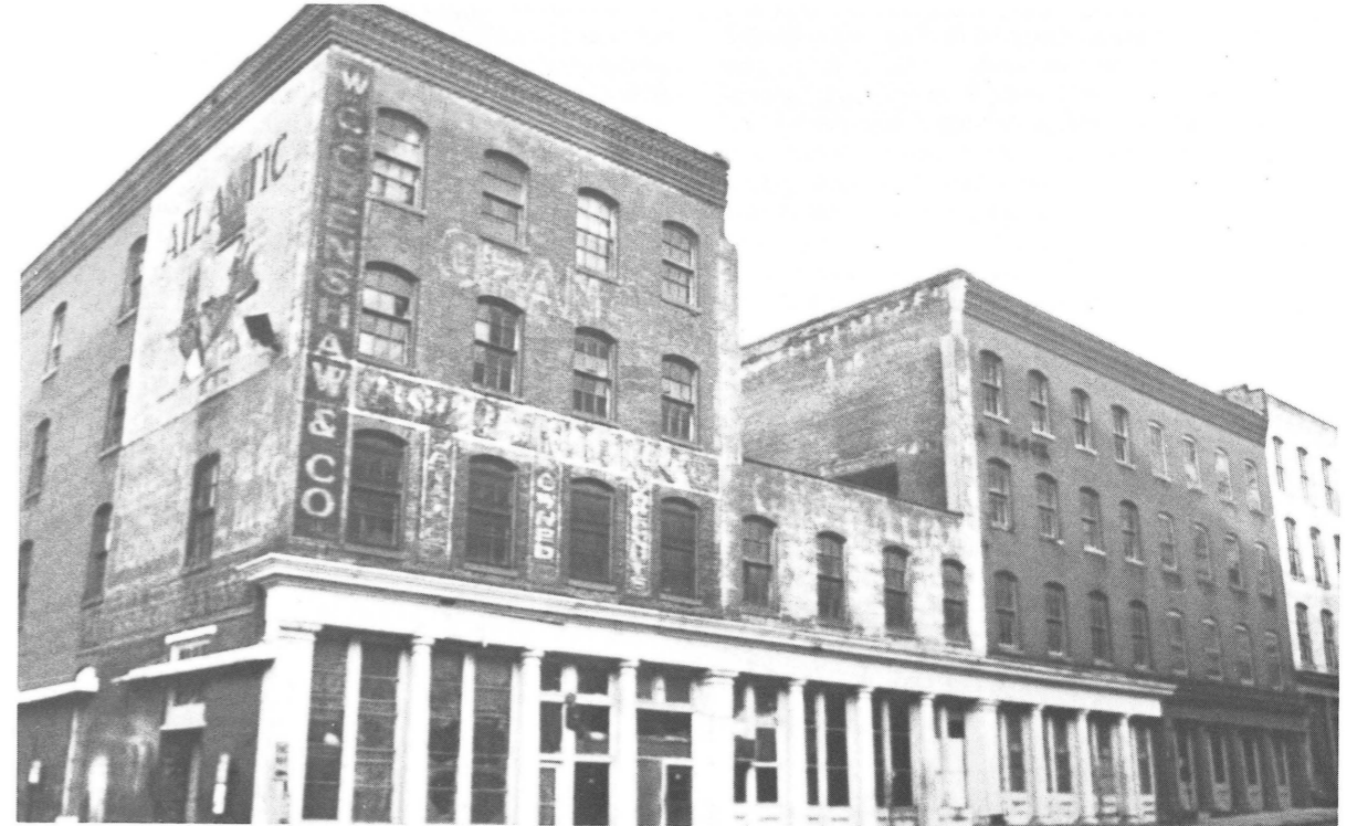
The Commercial Block before rehabilitation. Shockoe Slip Historic District, Richmond
