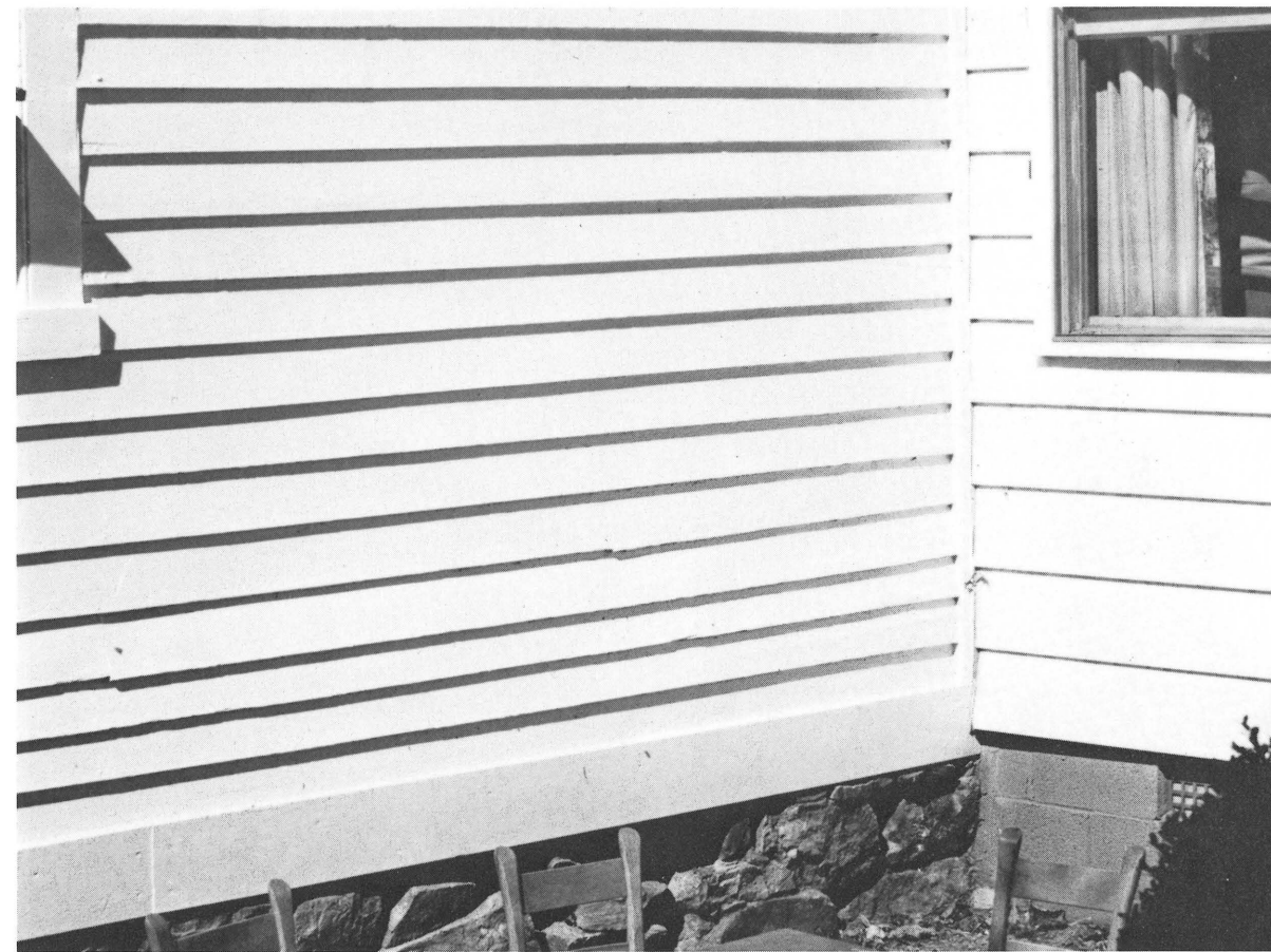
Plate Number Six: Original wood siding, at left, (after removal of metal siding) at intersection with metal clad wing showing difference in scale between the wood and the metal siding.
