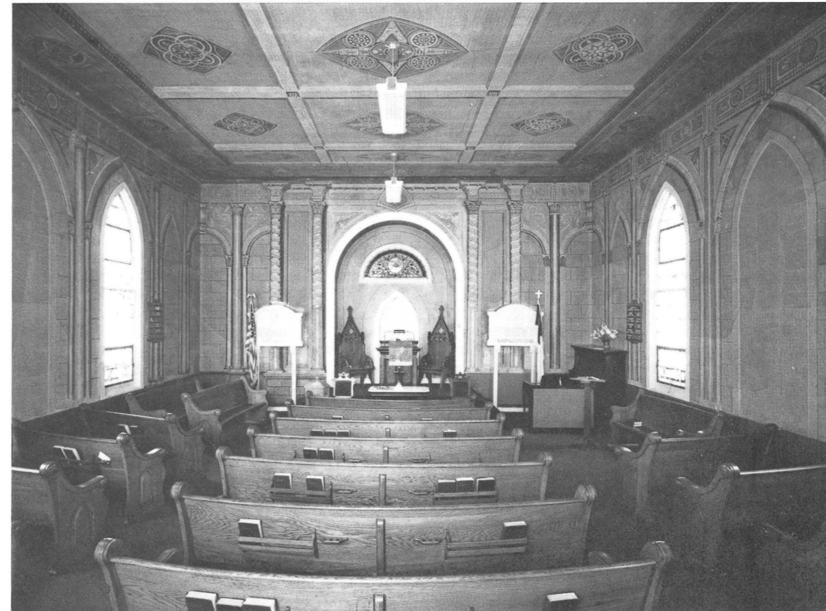
Plate Number Two: Interior of church in 1979 before restoration, showing advanced plaster cracking and Twentieth Century intrusions such as fluorescent light fixtures and marble memorial plaques.
