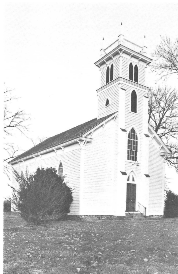
Plate Number Eight: Exterior of church in 1984 after restoration.
