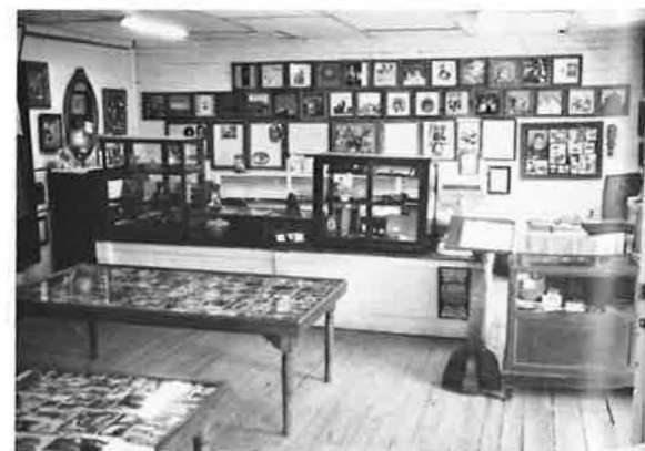
A. P. Carter Store, Scott County (interior).
