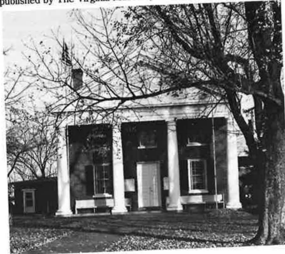
Goochland County Courthouse, from Architecture in Virginia, published by The Virginia Museum, Richmond, VA. 1968.
