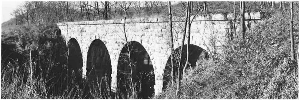
Valley Railroad Stone Bridge, adjacent to Interstate 81 in Augusta County. Credit: Virginia State Library
