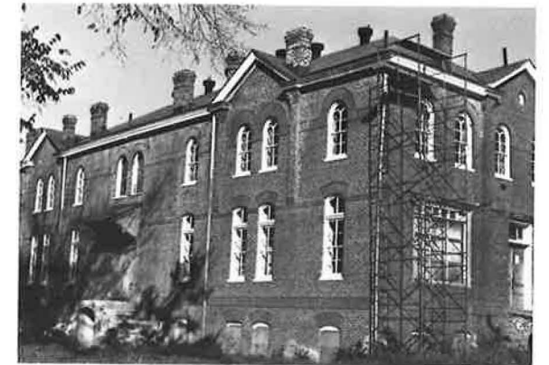
Main building of the Laurel Industrial School Historic District, Henrico County. Credit: Sara Amy Leach
