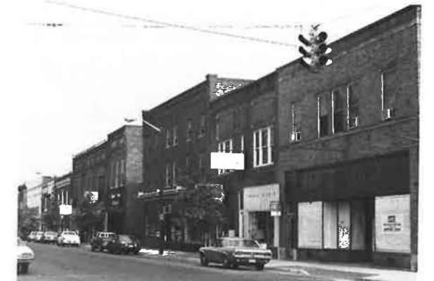
South side of Main Street in the Pulaski Historic Commercial District, Pulaski County. Credit: Charlotte Worsham
