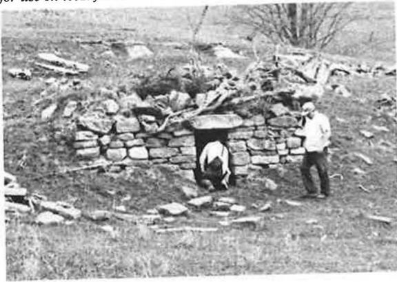
Abandoned lime pit at Burke's Garden. Such structures were constructed to burn blocks of limestone, converting them into lime for use on local farms.
