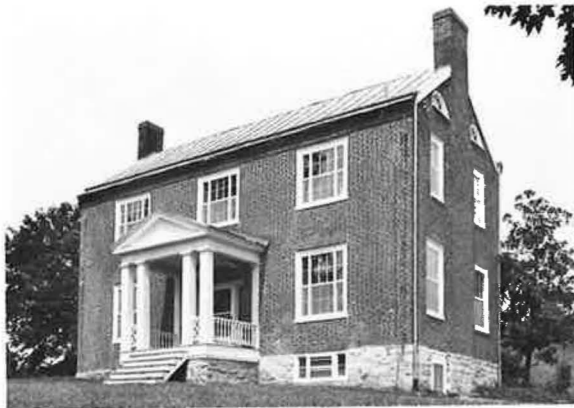
Locust Hill, Rockbridge County. Credit: Patrick Hinely
