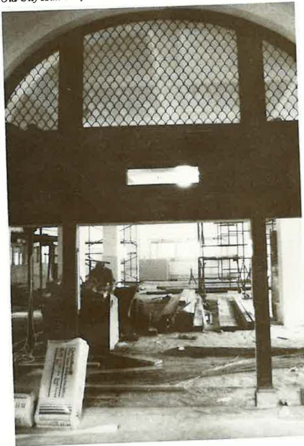
Old City Hall Norfolk. Atrium entry before rehabilitation.
