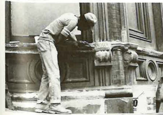
Brownstone repair at the Chesterman Place, 100 West Franklin Street, Richmond.
