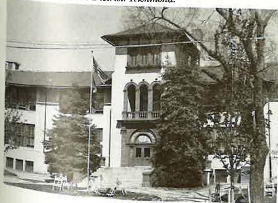
Ginter Park Elementary School at 3817 Chamberlayne Avenue, Ginter Park Historic District, Richmond.
