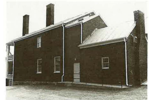
Willson Walker House, Lexington. Rear of building after rehabilitation completed.
