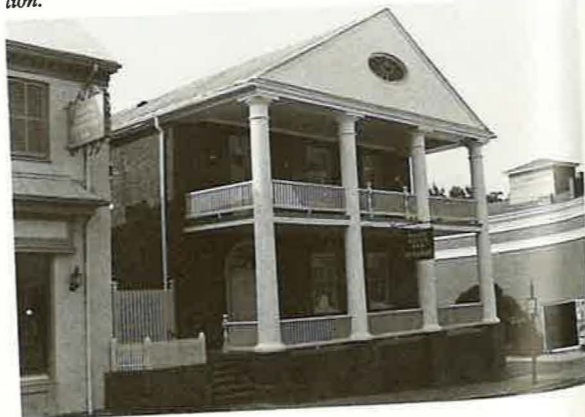
Willson Walker House, Lexington. Front elevation after rehabilitation.
