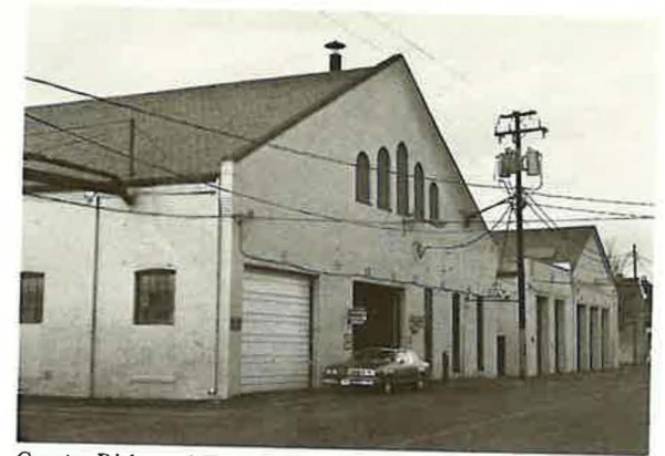
Greater Richmond Transit Company Bus Barns in the Fan Area Historic District Extension, Richmond.
