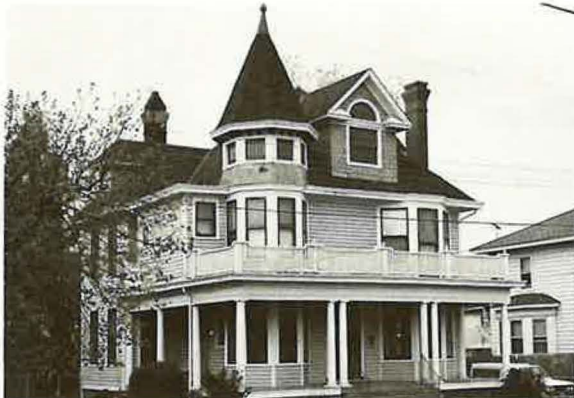
Harold Norton House in the North End Historic District. Newport News.
