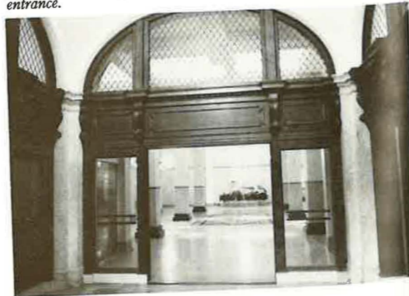
Atrium entry to Old City Hall, Norfolk, after completion of rehabilitation. View is looking into the new atrium which was the old mailroom. Existing screen has been restored and adapted for entrance.
