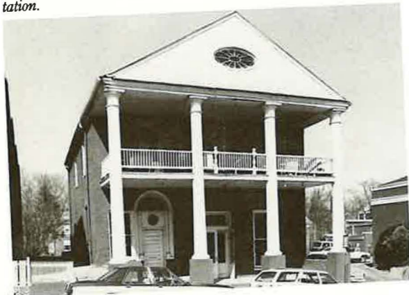
Willson Walker House, Lexington. Front elevation before rehabilitation.
