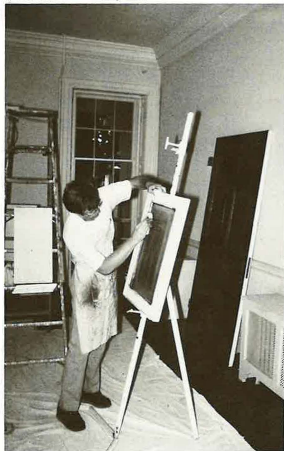
Exact replica patterns for graining are developed over many weeks of "trial and error" on test panels.
