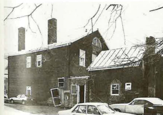
Willson Walker House, Lexington. Rear of building prior to rehabilitation.
