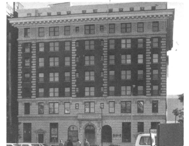
The Fairfax Hotel with the reconstructed cornice. Downtown Norfolk Historic District.
