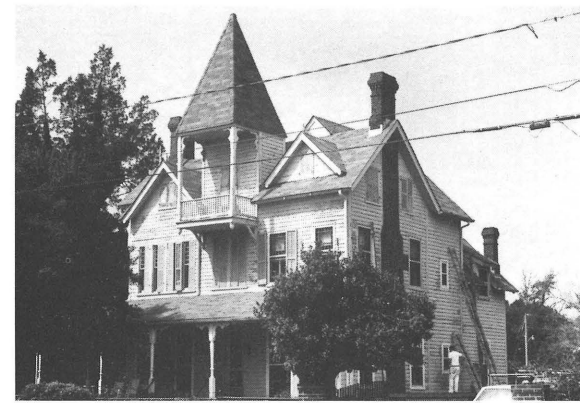
Bell House, Colonial Beach, Westmoreland County.
