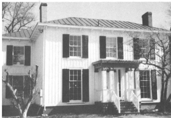
William Marien House, after rehabilitation.
