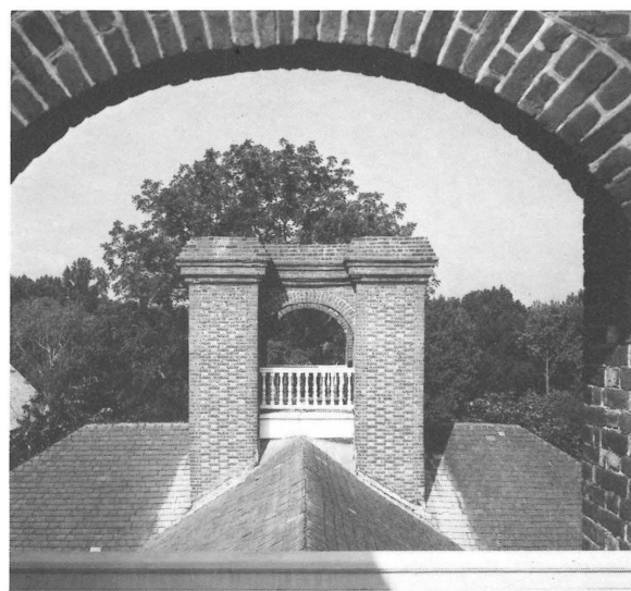
Stratford's unique chimney clusters. Credit: Historic American Building Survey
