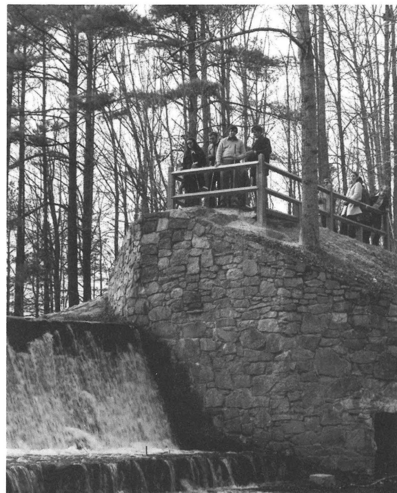
Pocahontas State Park in Chesterfield County, built in the 1930s, has interesting dams and roadways.
