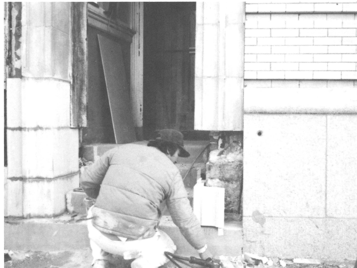
Rehabilitation work underway on the Fairfax Hotel, Downtown Norfolk Historic District.
