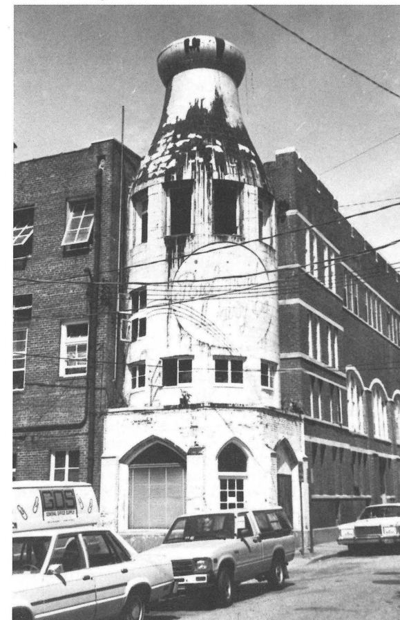
Broad Street Commercial Historic District, Richmond; the "Milk Bottle Building."
