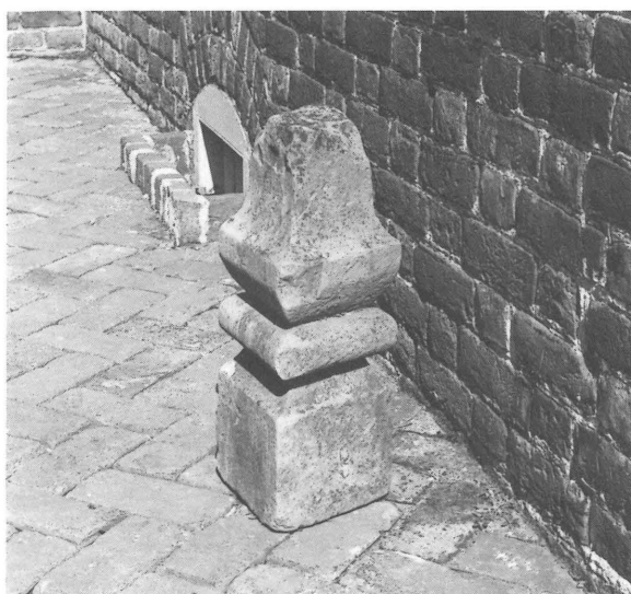
An original baluster recovered from the garden at Stratford. This formed the basis for the design of the exterior stair by Fiske Kimball.
