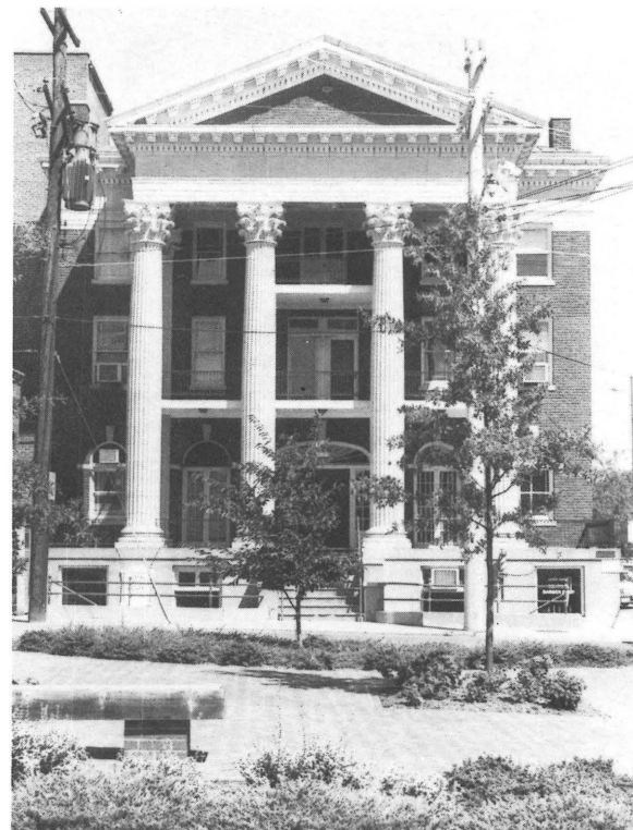
103 West Frederick Street, Staunton after rehabilitation of elaborate Colonial Revival facade.
