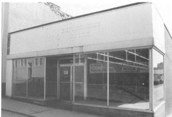
202 East Washington Street, before.
