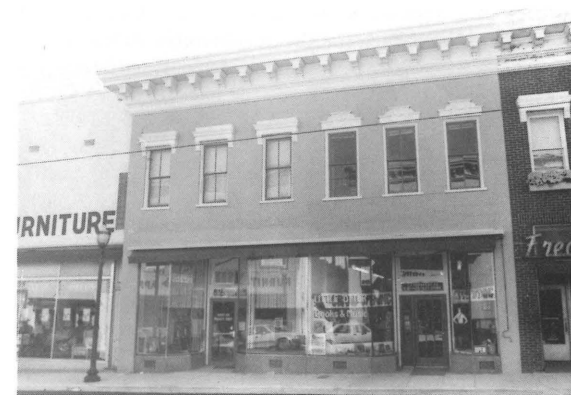
The same building after rehabilitation with paint cleaned off the windows, old signs removed, awning replaced, and a new paint scheme.
