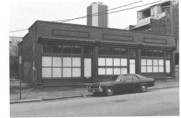
2-6 South 18th Street, Shockoe Valley and Tobacco Row Historic District, Richmond. After rehabilitation.
