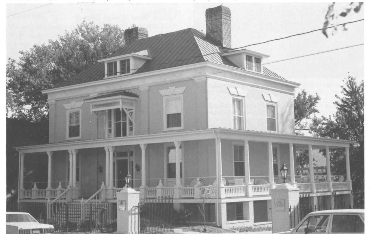
South Street Inn, Charlottesville, completion of rehabilitation with original porches replaced.
