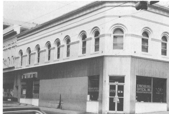
102-106 N. Bridge Street, Bedford. Before.
