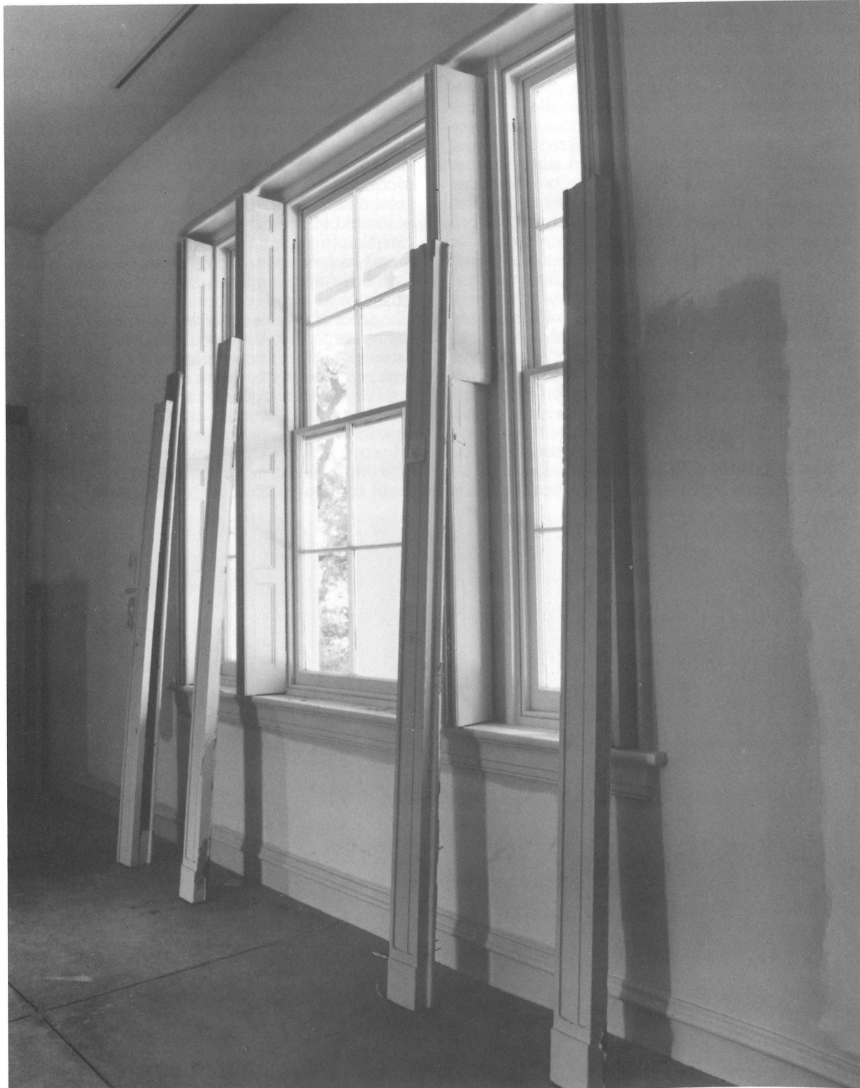
Katherine Wetzel, photograph, 1987, Window, Davis's Office. The recently discovered pieces of trim have been returned to their original locations for study, that will ultimately lead to the reconstruction of the windows to their wartime appearance. All window trim will be restored along with baseboards and doortrim.
