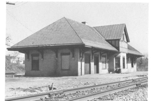
Norfolk-Southern Railroad Depot, Berryville Historic District, Clarke County.
