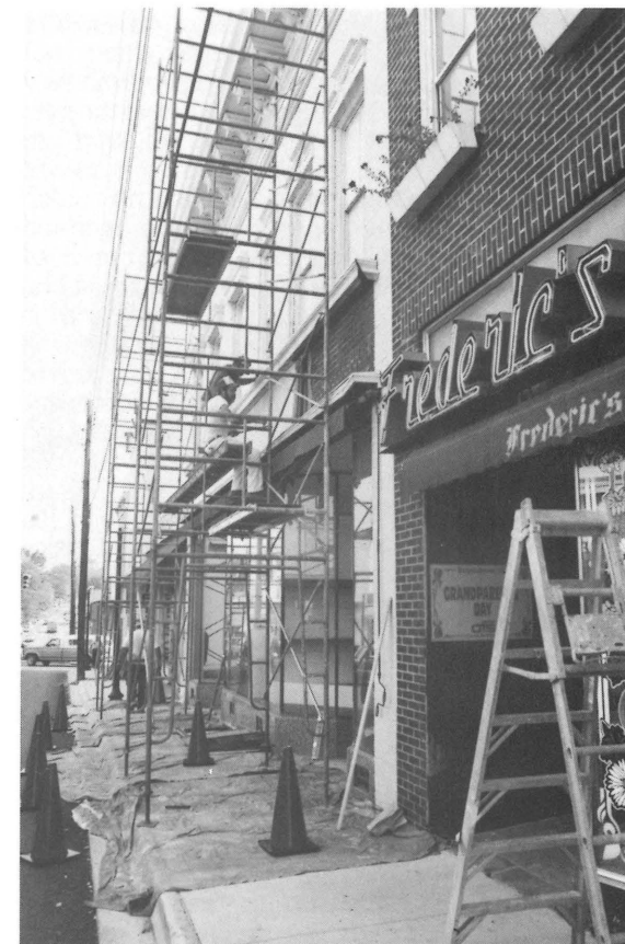
114-118 N. Bridge Street, Bedford during rehabilitation.
