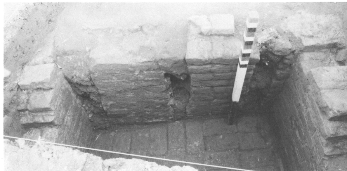
Bulkhead entrance discovered at Arlington Site.
