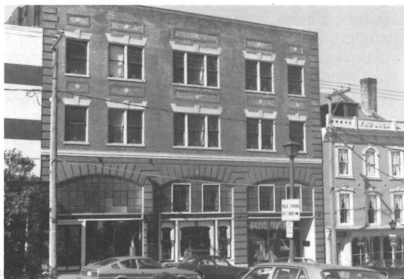
408-412 N. Sycamore Street, Petersburg. The facade has been cleaned and painted and new retail space created.
