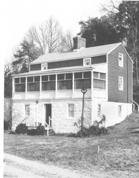
Lock Keepers House, Goochland County.
