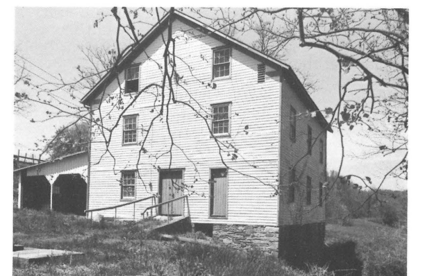
Mill in the Buckland Historic District, Prince William County.
