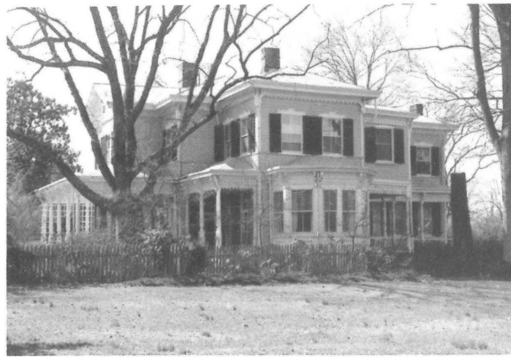
T.M.R. Talcott House at 1730 Buford Road, Bon Air Historic District, Chesterfield County.
