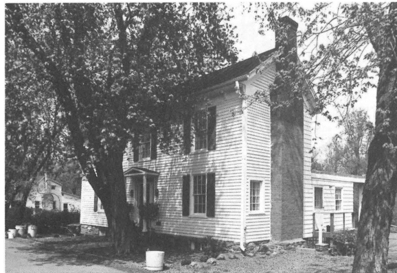
Buckland Historic District, Prince William County.
