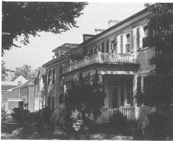
100 Block East High St., Charlottesville property subject to Charlottesville ordinance relating to demolition by neglect.
