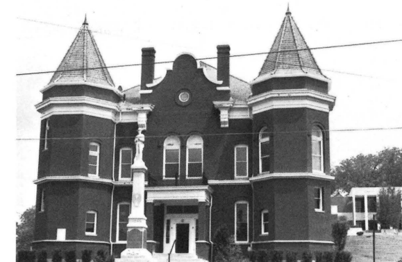
1908 Grayson County Courthouse, Independence, Grayson County
