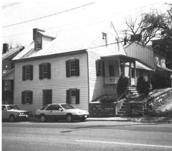
1115 First Street, S.W., Roanoke; after rehabilitation
