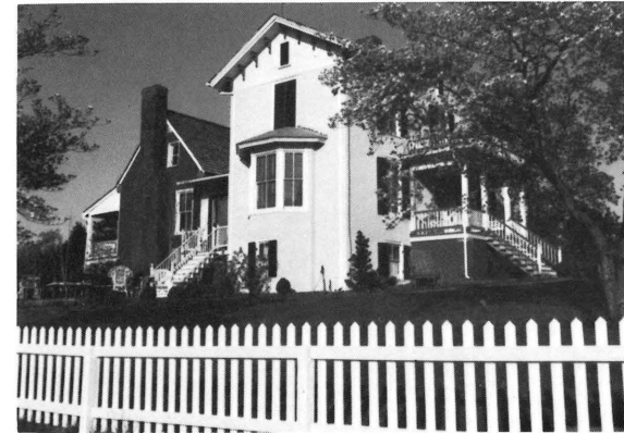
High Meadows, Scottsville, Albemarle County; after rehabilitation
