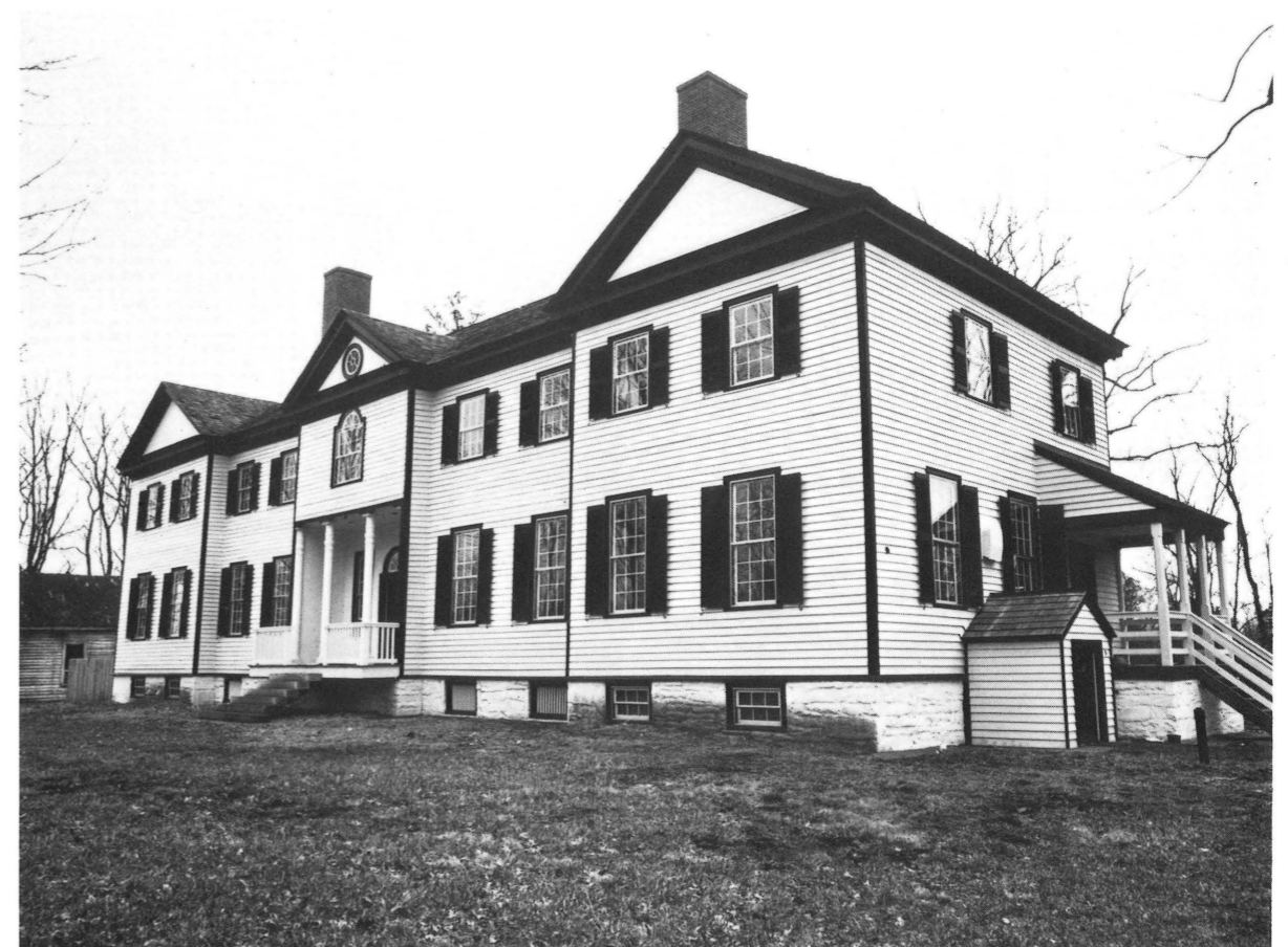
Farley, after rehabilitation
