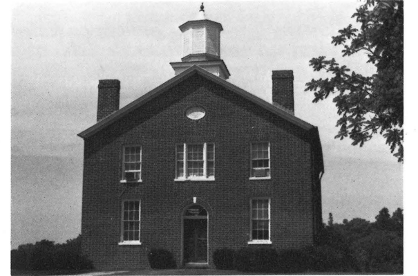
Brentsville Courthouse and Jail, Brentsville, Prince William County. Credit: Jan Townsend
