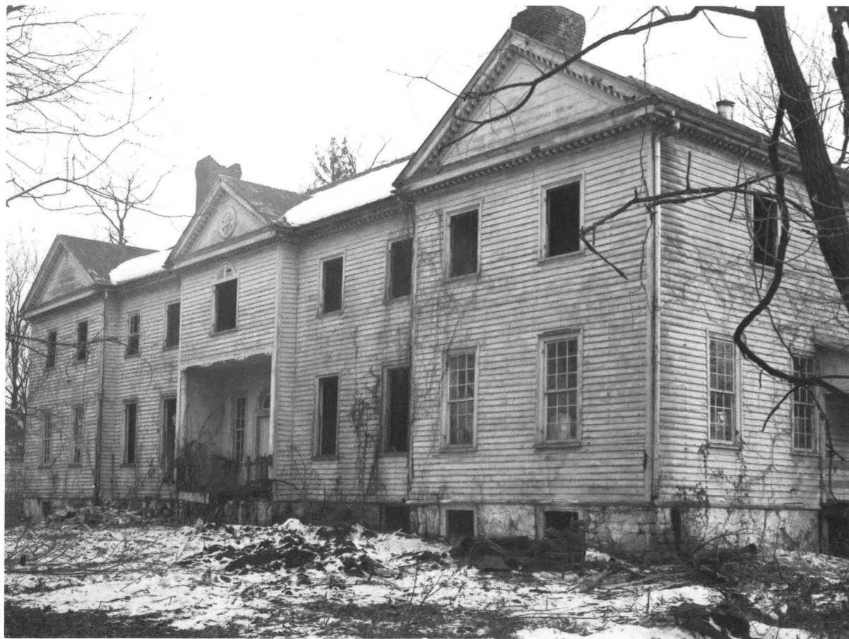
Farley, Brandy Station vicinity, Culpeper County; before rehabilitation
