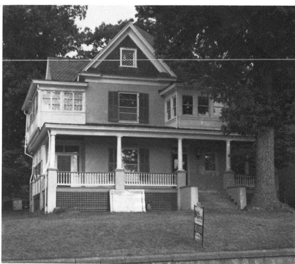
213-215 N. Augusta Street, Staunton; after rehabilitation
