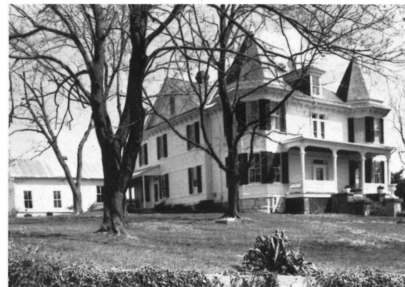
Campbell Farm, Lantz Mills, Shenandoah County, reflects the optimism that pervaded the post-bellum era in the Shenandoah Valley.
