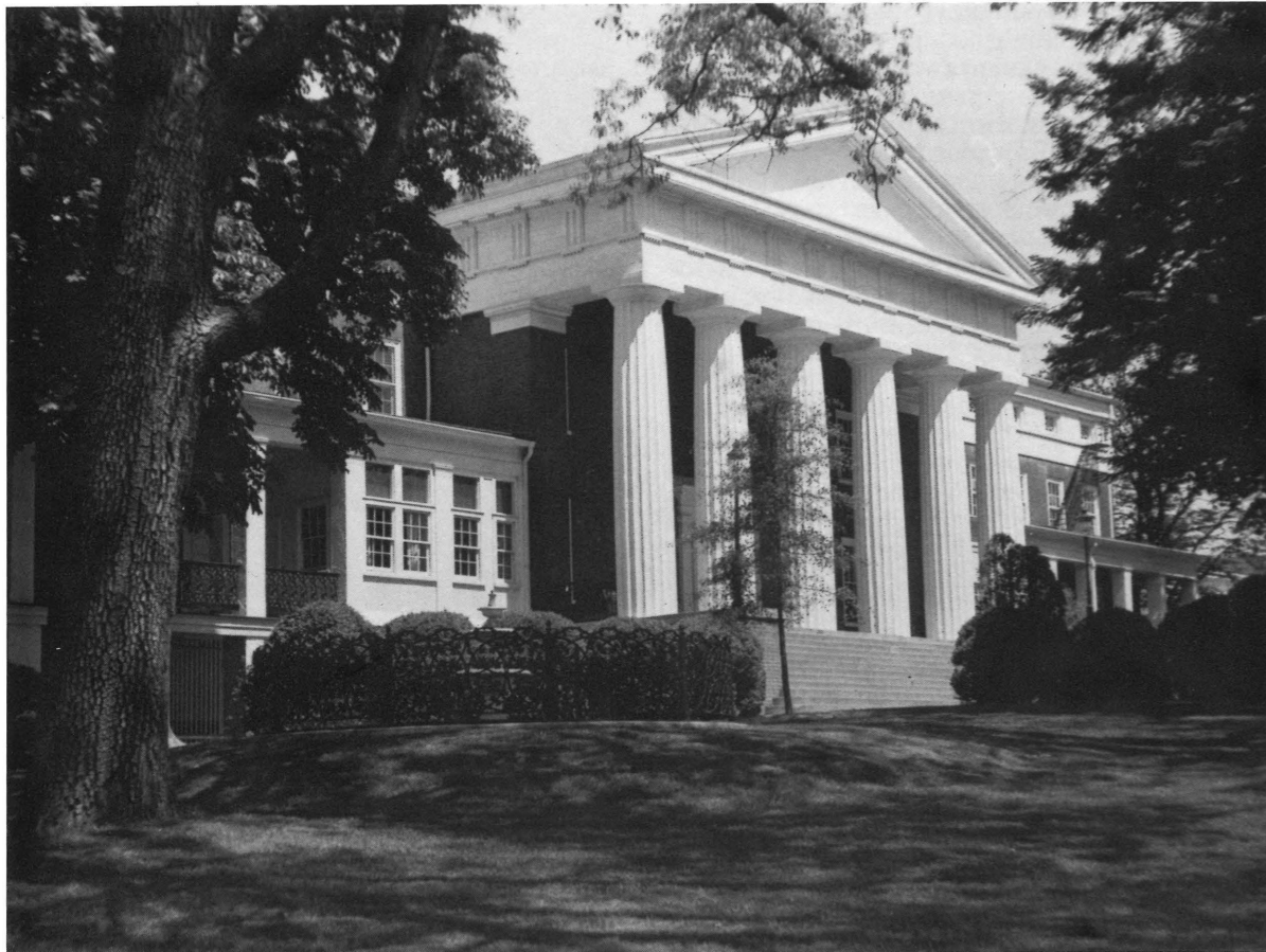
The survey recommends an enlargement of historic boundaries at the Virginia School for the Deaf and Blind in Staunton.
