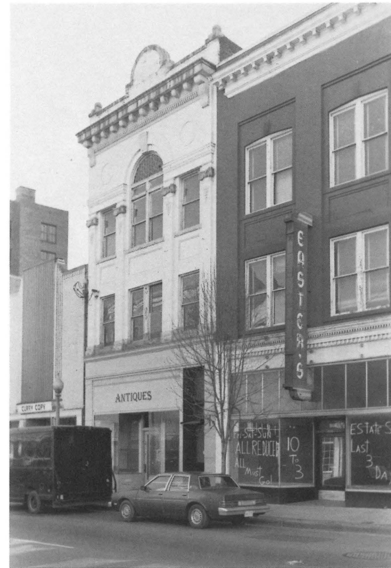
Campbell Avenue Properties, Roanoke.
