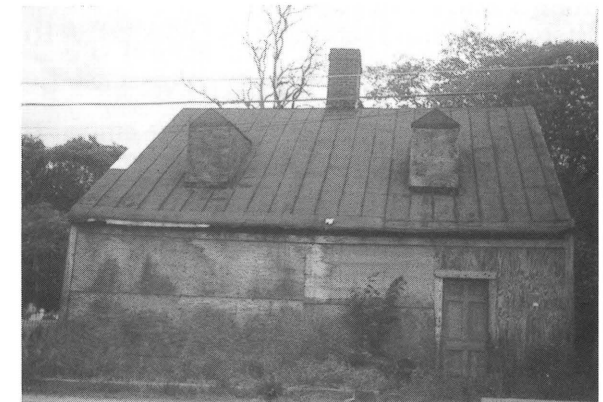
429-431 Cross Street, Petersburg Old Town Historic District, before rehabilitation.
