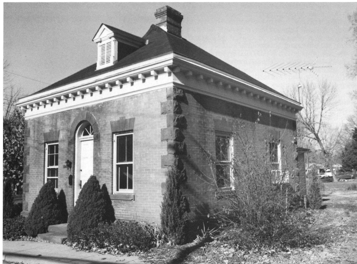
Portner Gate House, 9128 Portner Avenue, Manassas Historic District.
