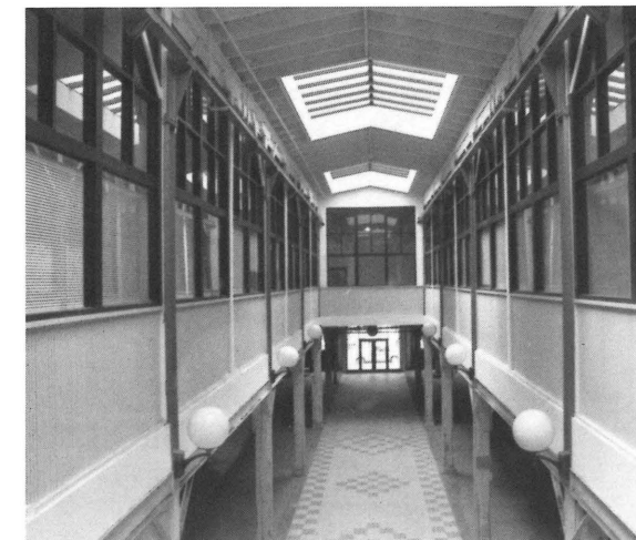
Superior Industrial Machine Complex, interior, following rehabilitation.
