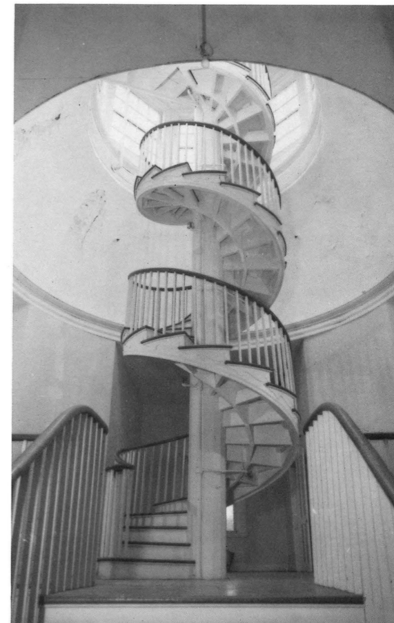
The interior staircase of Old Western State Hospital.
