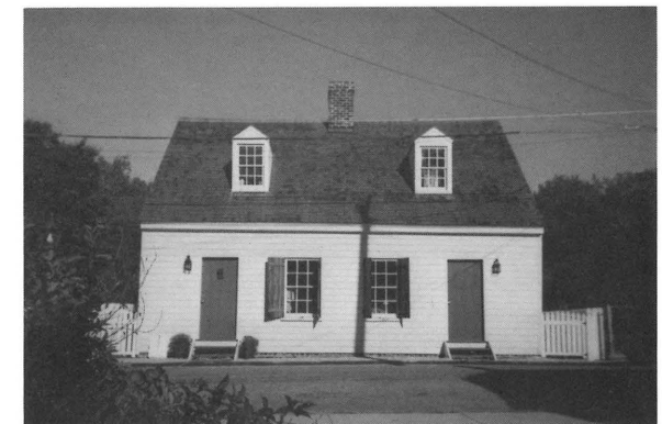
429-431 Cross Street after rehabilitation.
