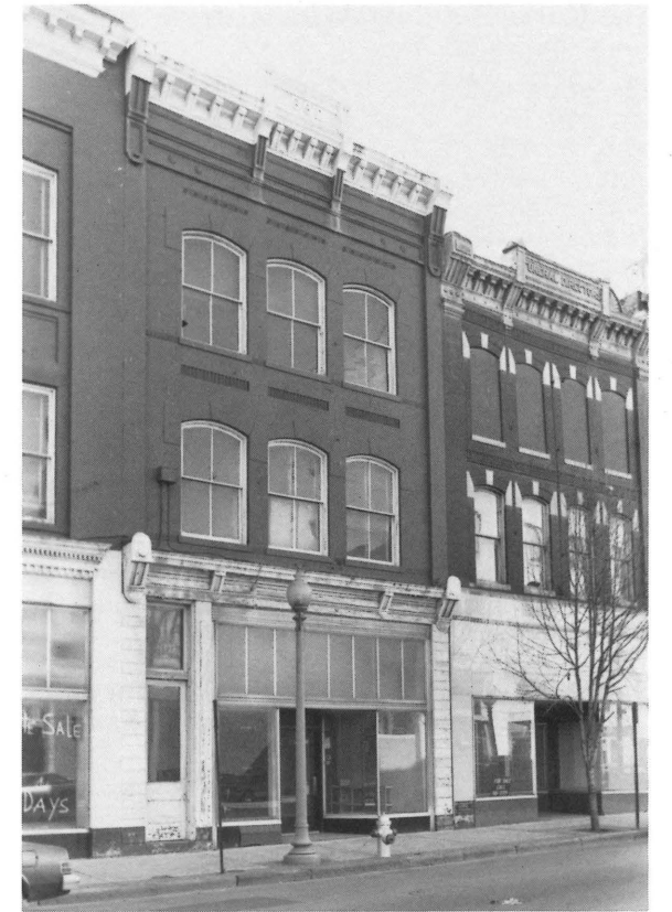
Campbell Avenue Properties, Roanoke.
