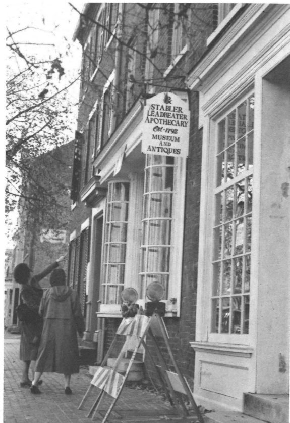
Repairs to windows, roof and building structure are in progress at the Stabler-Leadbeater Apothecary Museum in Alexandria.
