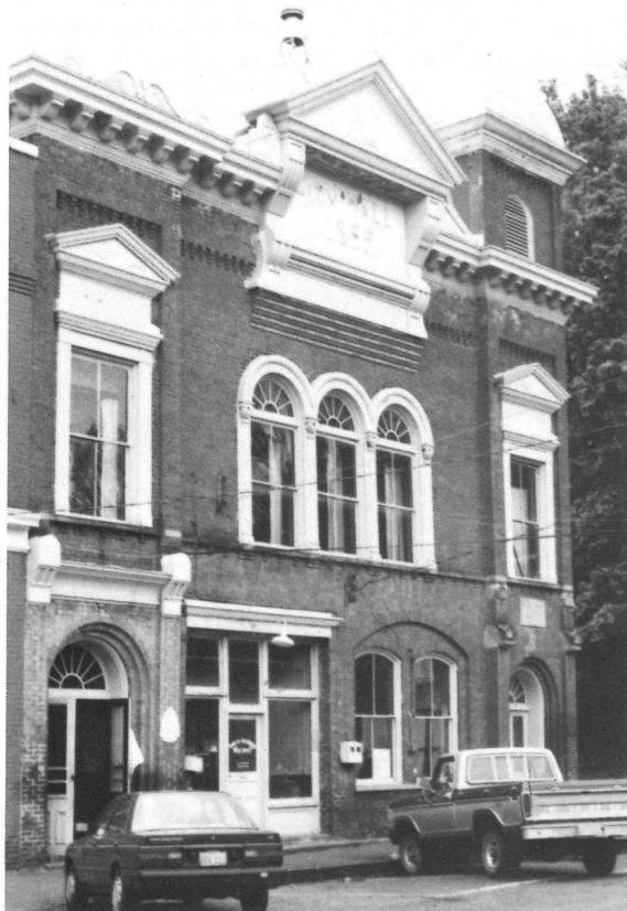
Threatened Properties Grant Funds have been used to make roof repairs to the Pocahontas Opera House in the town of Pocahontas in Tazewell County.
