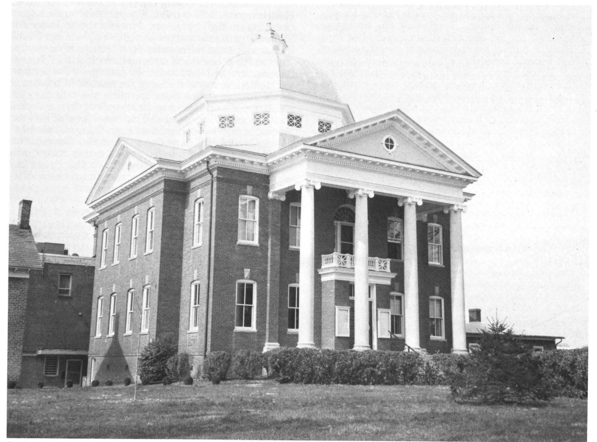
Louisa County Courthouse.
