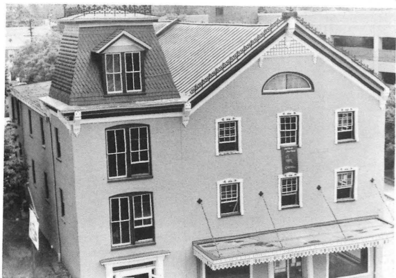
Preservation of Historic Winchester's rehabilitation of the Kurtz Building for use as a cultural center is nearing completion.
