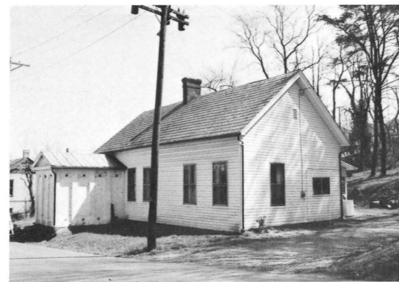
The office and vault of the Bertha Zinc and Mineral Company in the Pulaski South Historic Residential and Industrial District.
