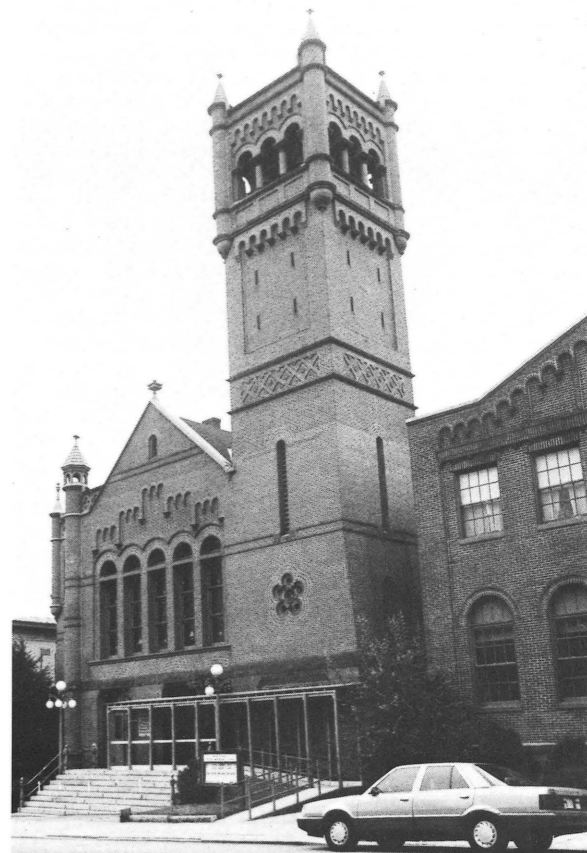
Main Street Methodist Church, Danville.
