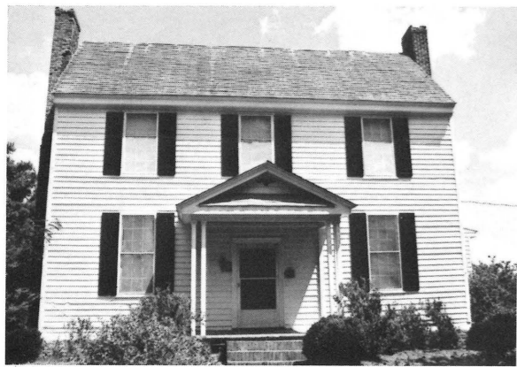
West facade of Rose Bower, Dinwiddie County.
