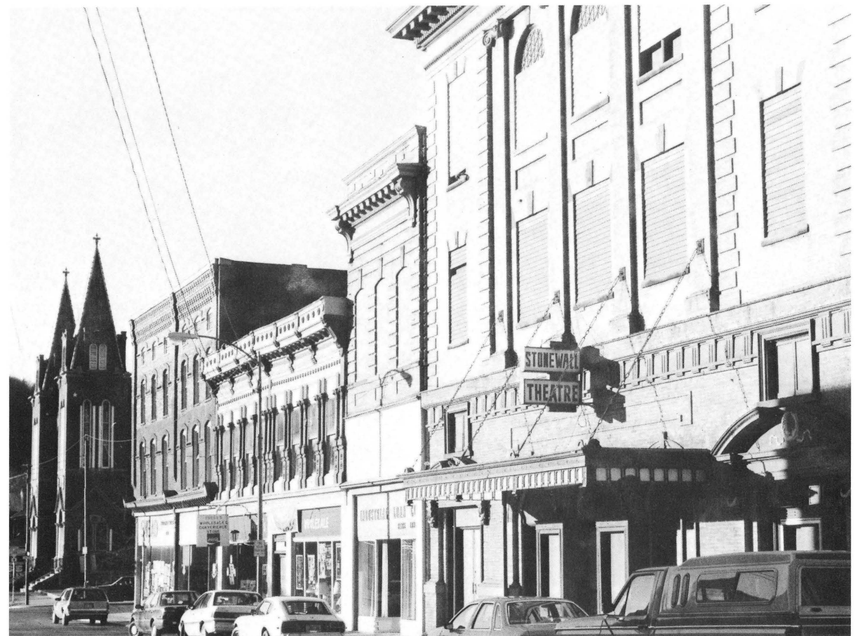
The 500 block of Main Street, Clifton Forge Commercial Historic District.
