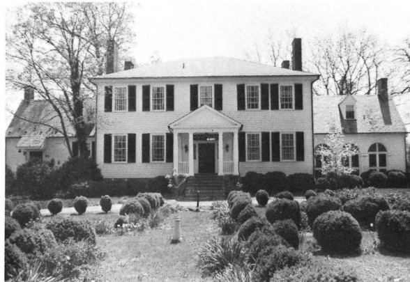
Rear elevation of the residence at Woodlawn, King George County.
