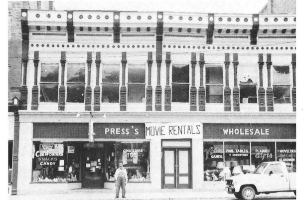
Carpenter, Moody & Company Building, 504 Main Street, Clifton Forge Commercial Historic District.
