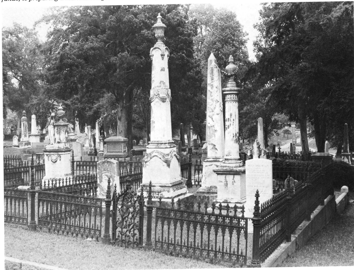
Registration calls special attention to significant structures or districts within a jurisdiction. Petersburg, using 1991 CLG funds, is preparing a National Register nomination for Blandford Cemetery. Credit: Sergei Troubetzkoy.
