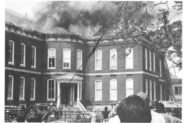
The Stonewall Jackson School in Richmond suffered considerable damage during a fire on April 24, 1990.
