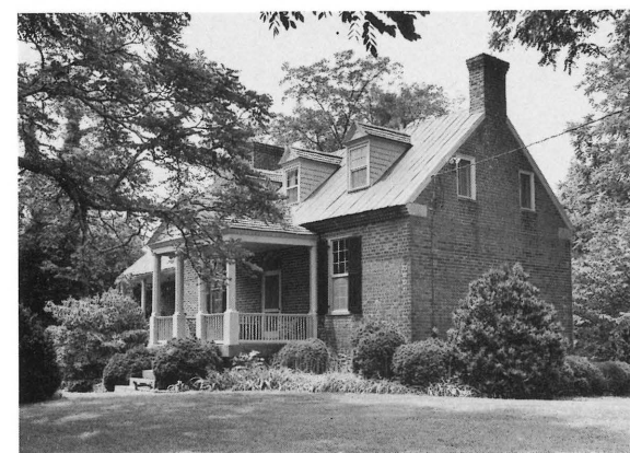
Hope Dawn, in Bedford County, illustrates high standards maintained by builders of even modest homes in remote areas.
