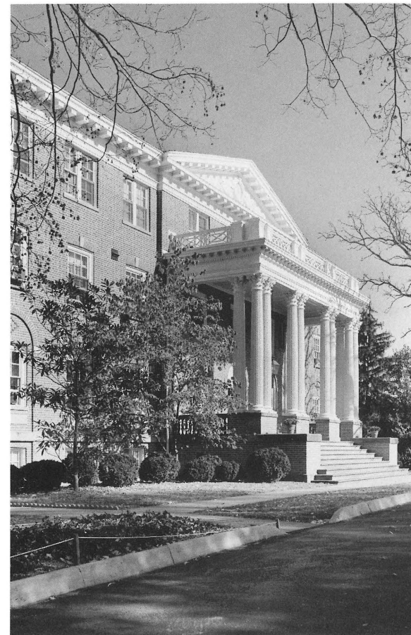
Virginia Episcopal School, City of Lynchburg.
