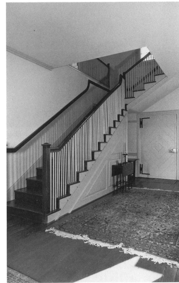
Interior of Grove Mount shows well-preserved Federal detailing.
