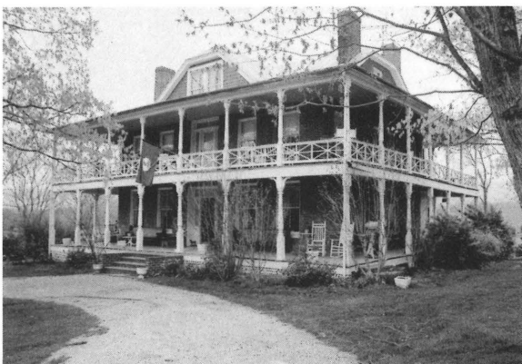
Rockbridge Inn, Rockbridge County
