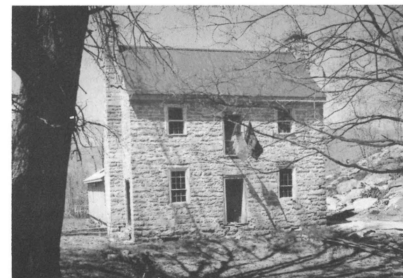
Scott-Walker House, Smyth County
