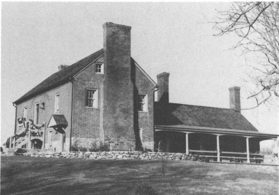
The McFadden House in the Kennedy-Wade's Mill Historic District, Rockbridge County
