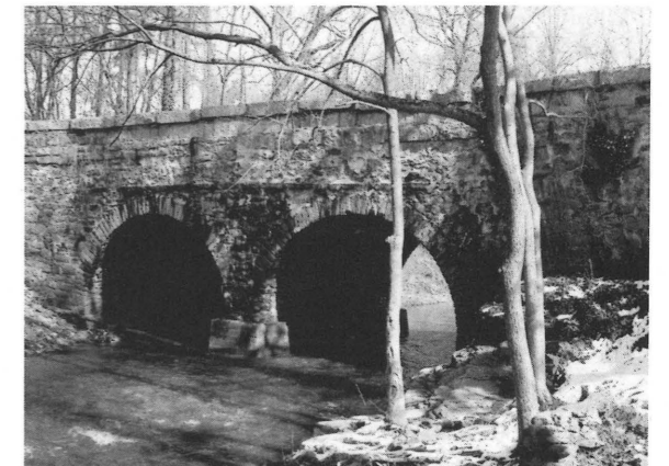
Bridge at Falling Creek, Chesterfield County
