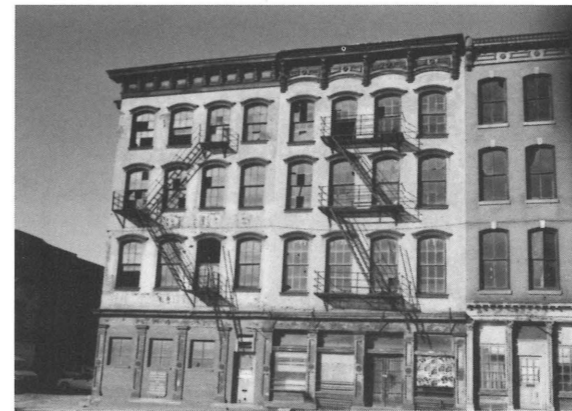
8-10 South 14th Street, City of Richmond, before rehabilitation.
