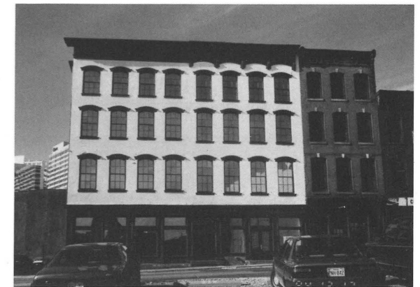
8-10 South 14th Street with the storefront rebuilt and existing ironfront remaining.
