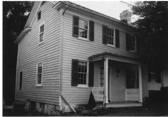
11 East Loudoun Street after renovation was completed.
