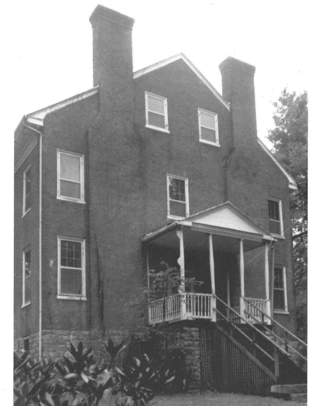
Brook Hall restored.
