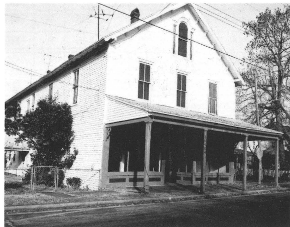
James Brown Dry Goods Store after work was completed.
