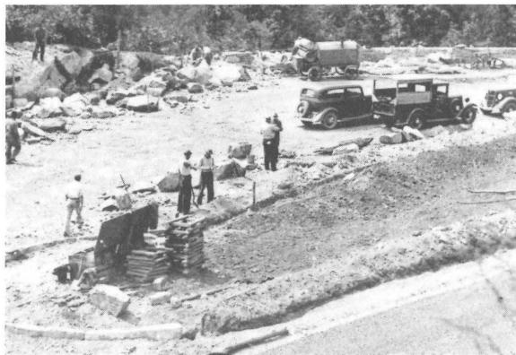
Skyline Drive under construction in the 1930s.
