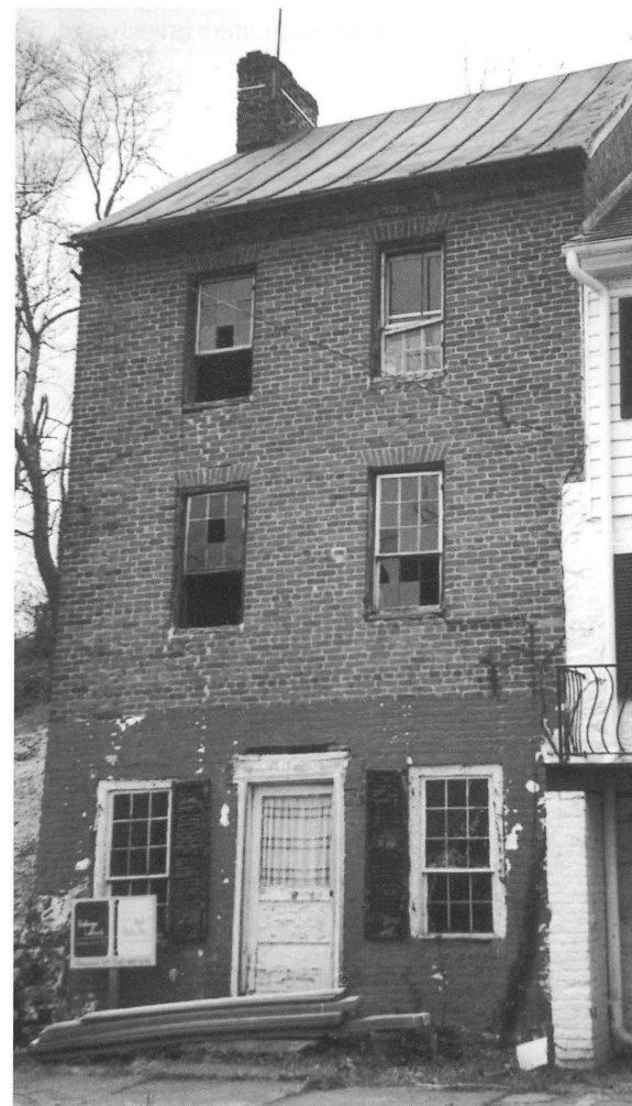
Janney-Coates House, Waterford – Before historic rehabilitation
