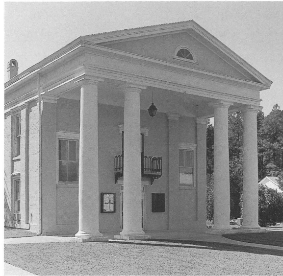
Dinwiddie County Courthouse, Dinwiddie County
