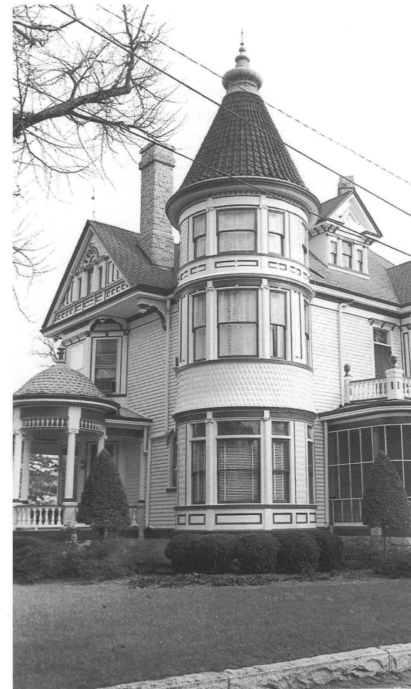
P. D. Gwaltney, Jr., House, Town of Smithfield
