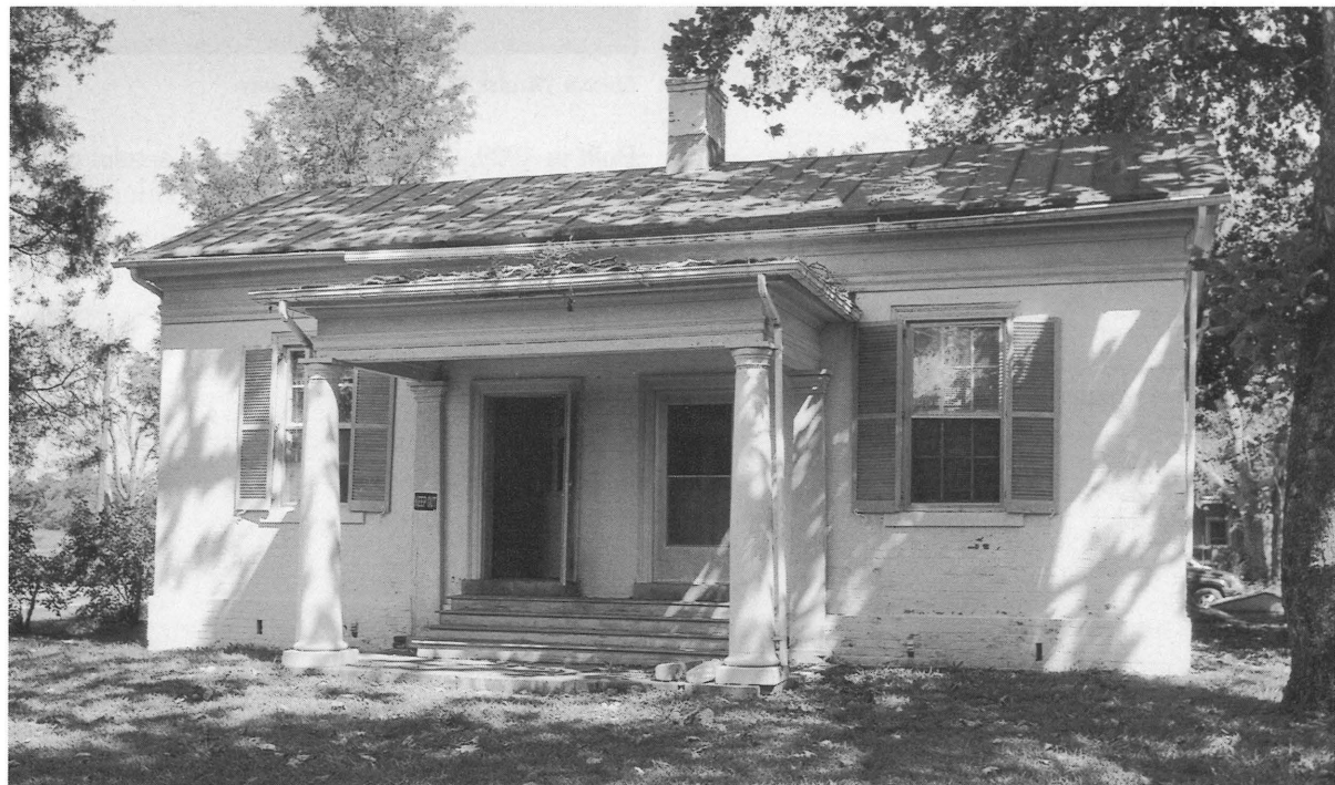
Old Prince Edward County Clerk's Office, Prince Edward County
