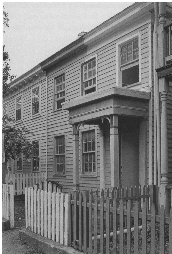
314 S. Pine Street, Oregon Hill Historic District, City of Richmond
