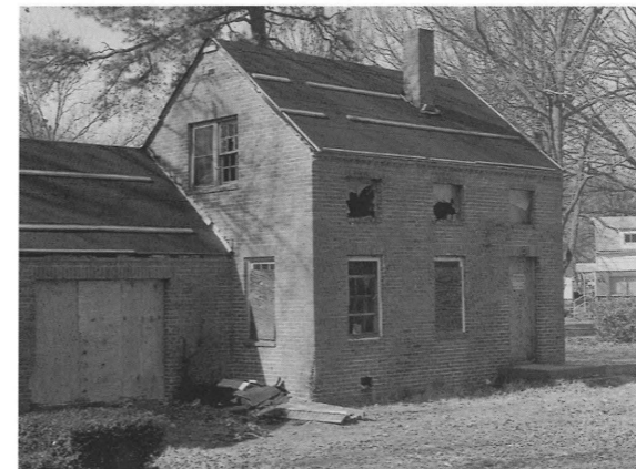
57 Mary Peake Boulevard, Aberdeen Gardens Historic District, City of Hampton
