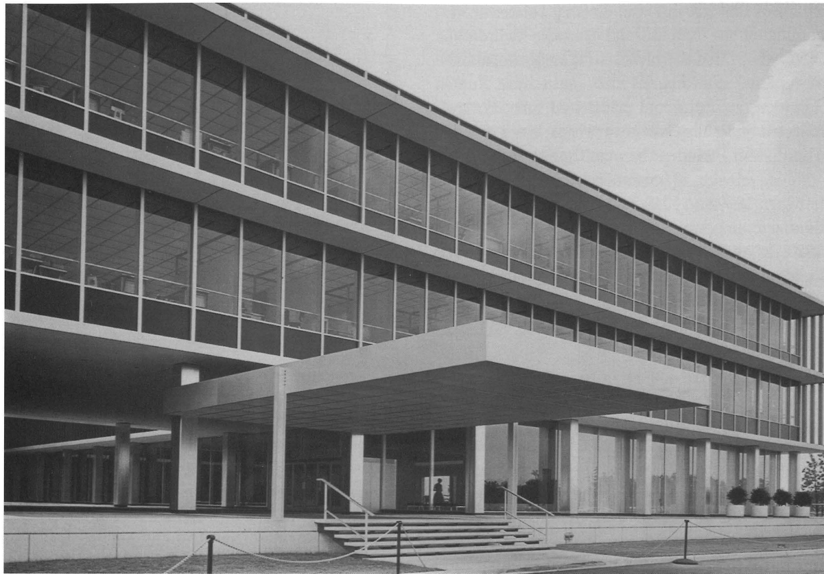
Reynolds Metals Company International Headquarters, Henrico County
