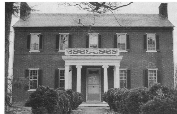
Andrew Johnston House, Giles County
