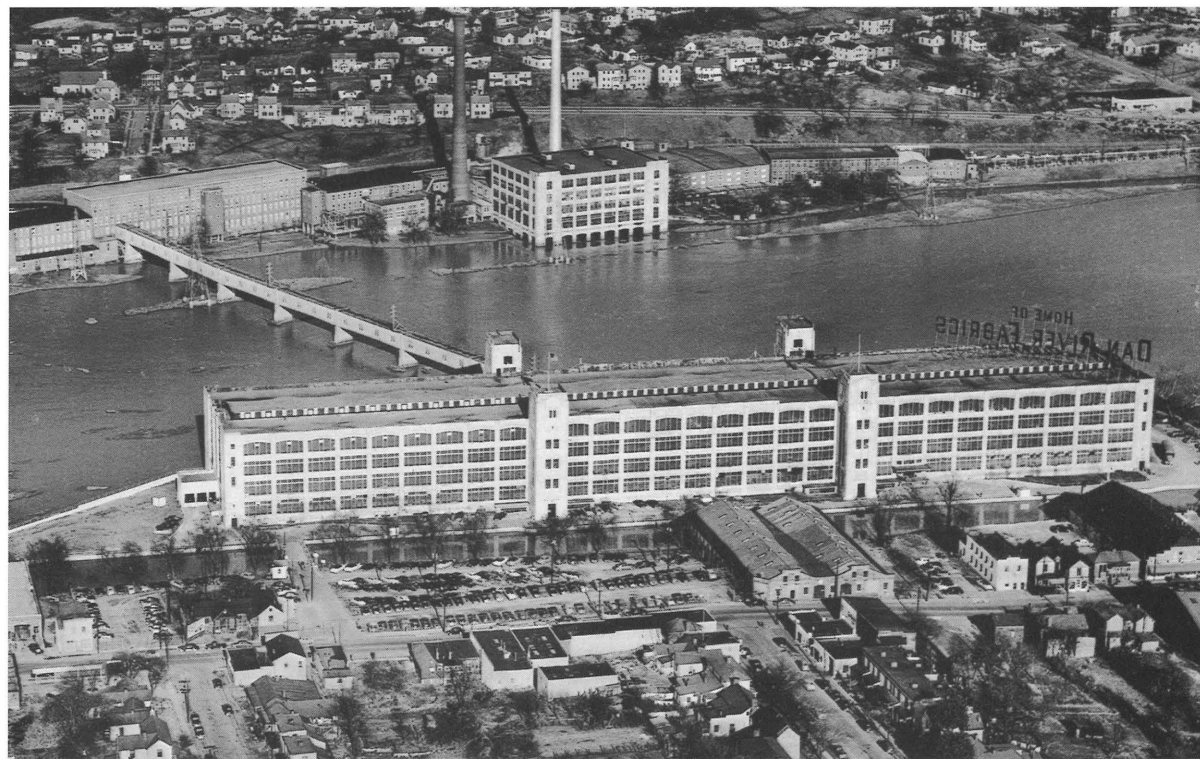
Dan River Inc. Riverside Division Historic District, City of Danville, (p. 16)
