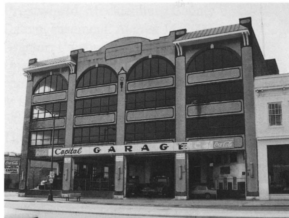
Capital Garage, Richmond, before rehabilitation
