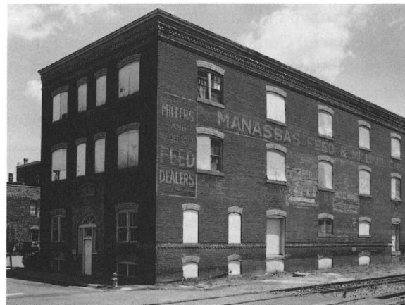
Hopkins Candy Factory Building
