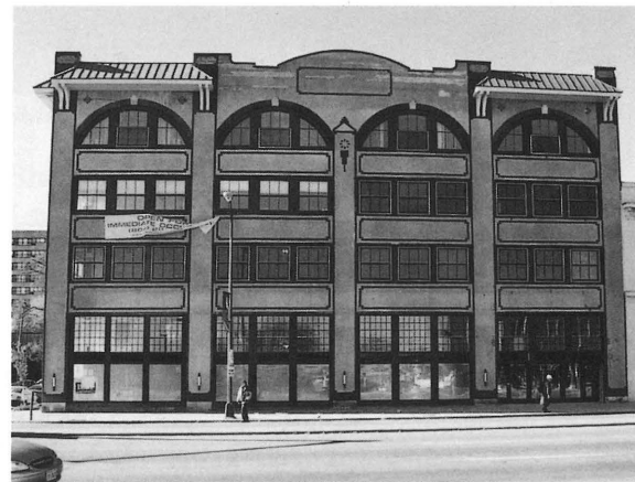
After rehabilitation as loft apartments
