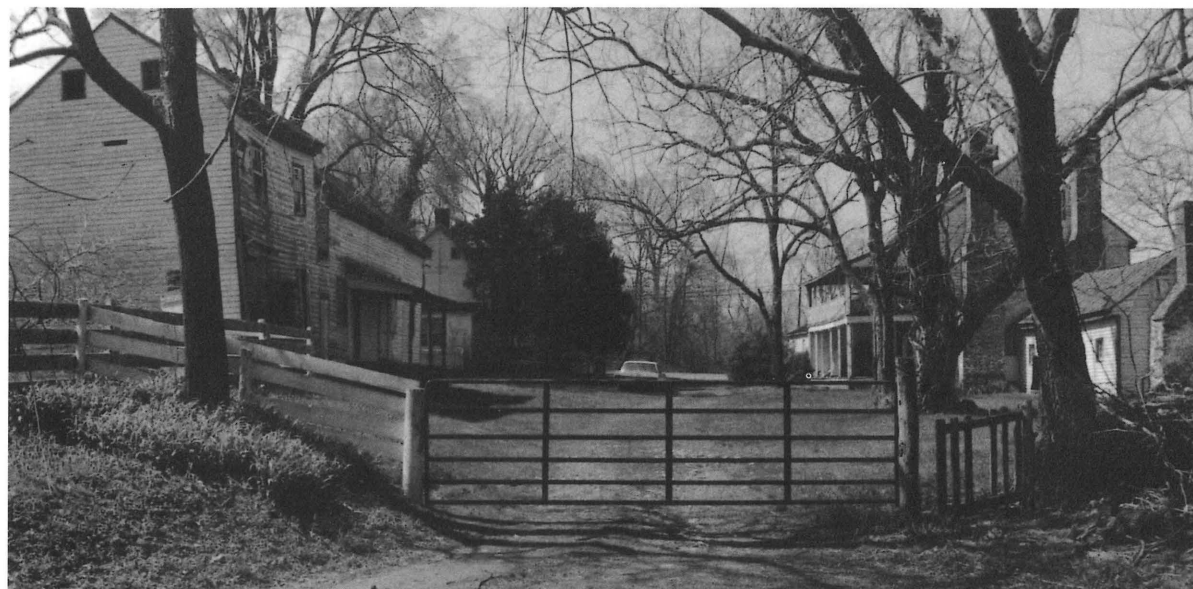
James City Historic District, Madison County
