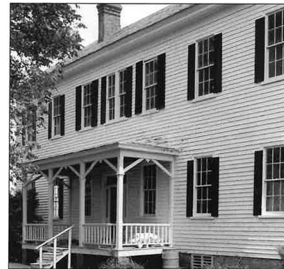
Almshouse Farm at Machipongo
