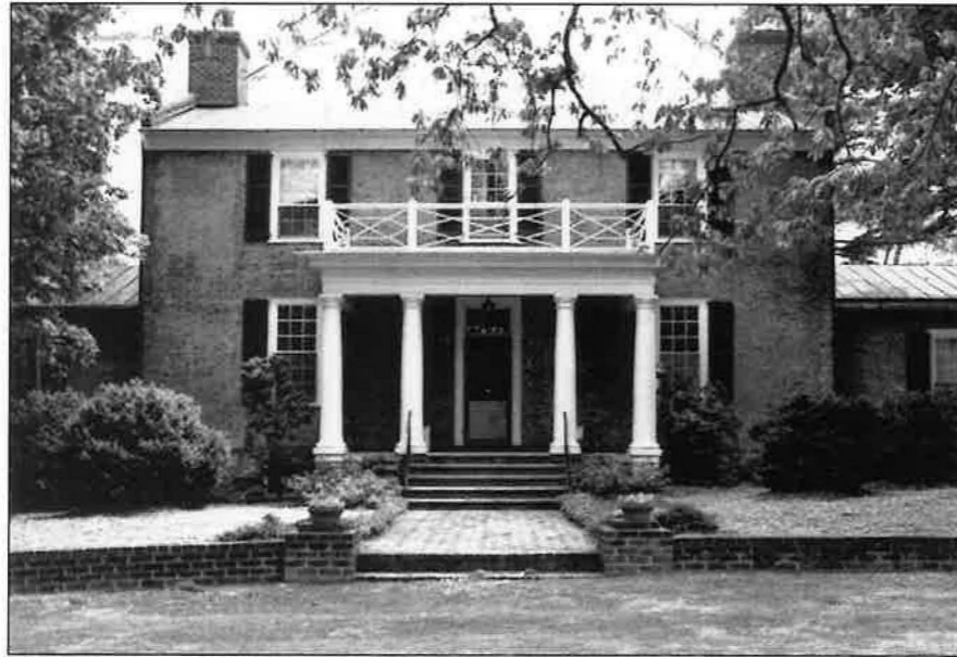
Montebello, City of Charlottesville
