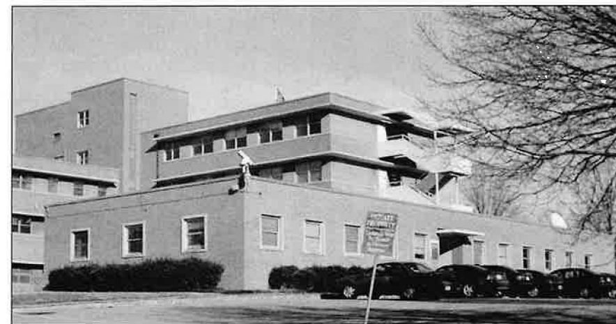
Burrell Memorial Hospital, City of Roanoke
