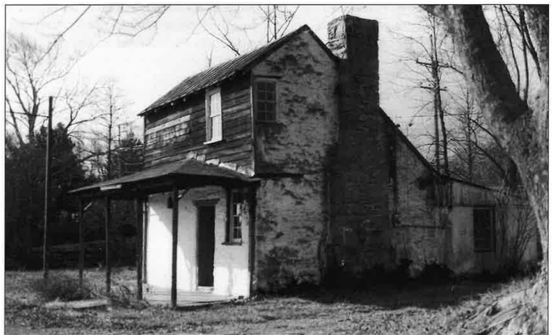
Tollhouse, Rappahannock County
