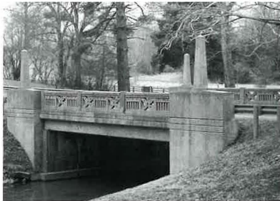
Appomattox River Bridge
