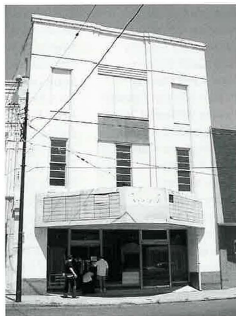
Danville's North Theater before restoration: The building was constructed circa 1900 and converted to a theater in 1947, with architectural modifications at the time that incorporated stylized Art Deco elements, the most prominent being the building's stucco façade.
