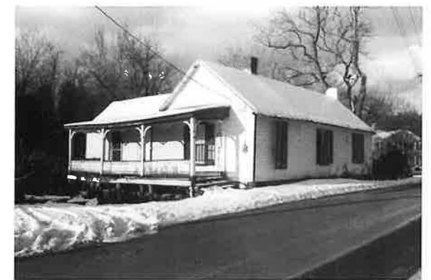
Lexington & Covington Turnpike Tollhouse
