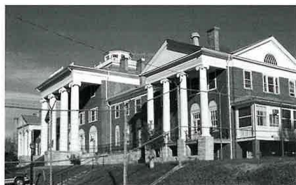
The south annex building at Western State was built by master mason William B. Phillips, who had worked for Thomas Jefferson at the University of Virginia.
