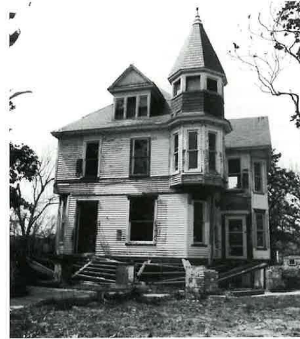
The Chandler House during renovation in 2004, without its wraparound porch
