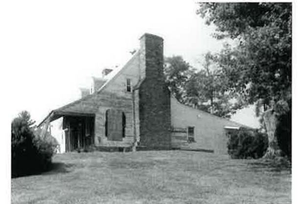
The former tavern-dwelling at Yew Hill during renovation
