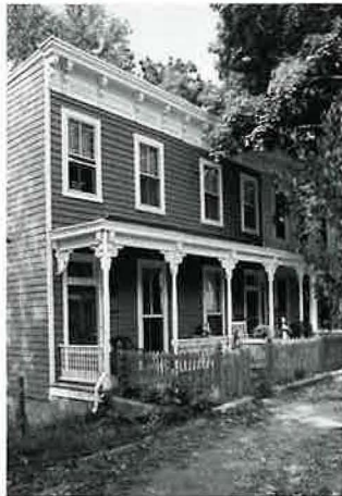
608 & 610 South Laurel Street
