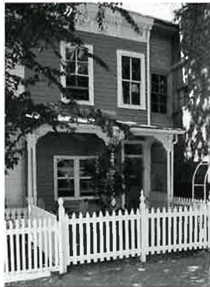
402 South Laurel Street
