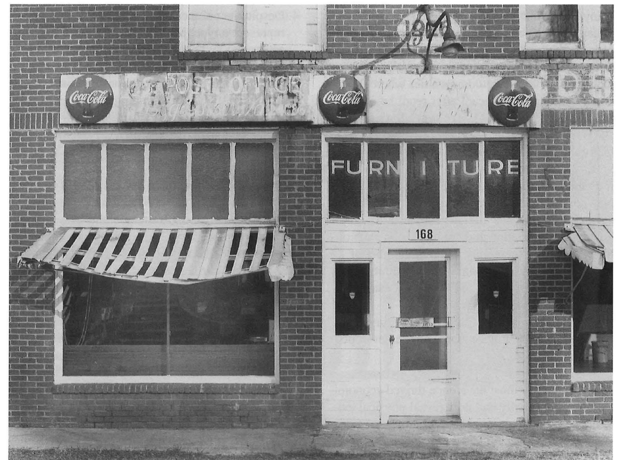
Signs on Gladys Dowdy's store in Eggleston show its previous incarnations. Eggleston was once the home of Eggleston Springs Resort and an important railroad depot for trade throughout Giles County. Upon its owner's death, Eggleston's general store closed, leaving a sleepy town with just a post office to attract residents to its downtown. (Photo: Kirsten Sparenborg, 2002)
