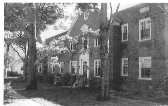
Lock Lane Apartments
