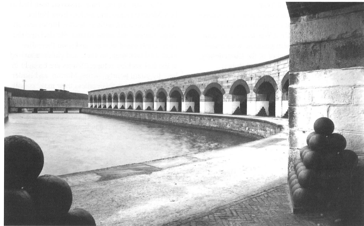
The magnificent casemated Water Battery was one of the defining architectural features of Fort Monroe. The water battery is a unique design not found in other American forts. Originally 40, 42-pounder sea-coast guns were mounted in the casemates. Casemate number 40 was a traditional rendezvous for young couples. Unfortunately the Water Battery was demolished in 1901. (Courtesy of Hampton History Museum)
