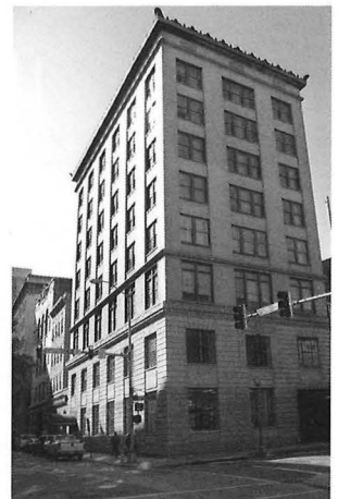
State & City Building
