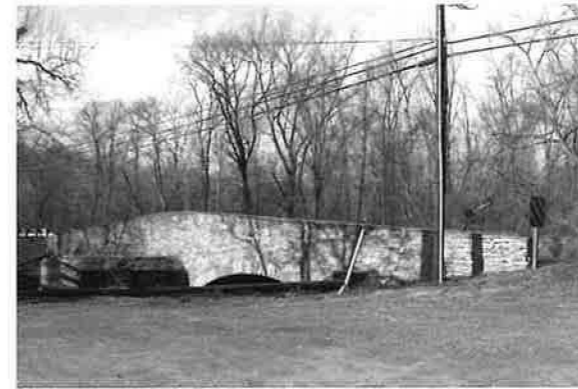
Little River Turnpike Bridge
