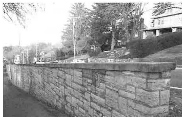
WPA-built bluestone wall in Old Town HD
