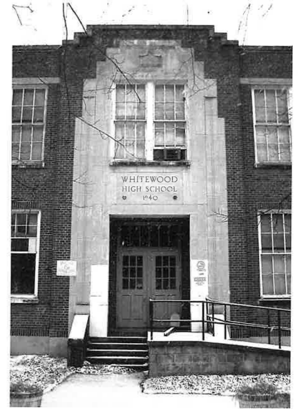
Whitewood High School, main entrance
