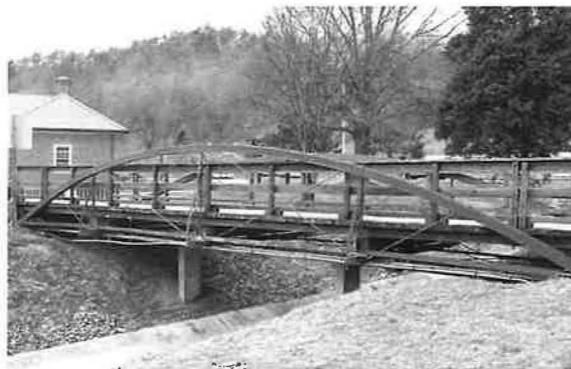
Bowstring Truss Bridge
