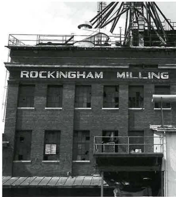
An enticing, dusty old building in Harrisonburg. The Rockingham Milling Company was established in 1919 and first appeared on the Sanborn map of 1924. Employing steel roller milling equipment likely purchased from firms supplying the huge milling industry in the upper Midwest, RMC and mills like it in Staunton and elsewhere displaced the ubiquitous stone grist mills [e.g. see p. 23] that had been dominant in the Shenandoah Valley in the 18th and 19th centuries. (Author photo)
