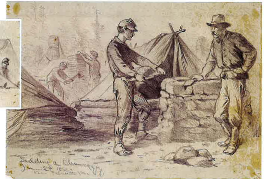
On January 15, 1863, artist Edwin Forbes sketched this hut near Camp Starvation. Having leveled the top of the stone firebox, the soldiers probably finished their chimney with clay-daubed logs or barrels. (Library of Congress)
