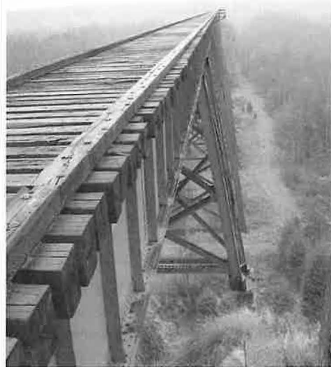
Current High Bridge
