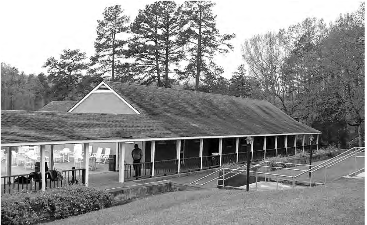
Cedar Crest Conference Center, Twin Lakes SP
