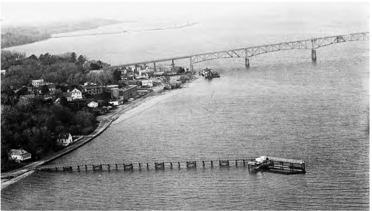
An aerial view of the cofferdam that was erected during the archaeology on the Yorktown Shipwreck site that is listed in the Virginia Landmarks Register and National Register of Historic Places. (DHR)
