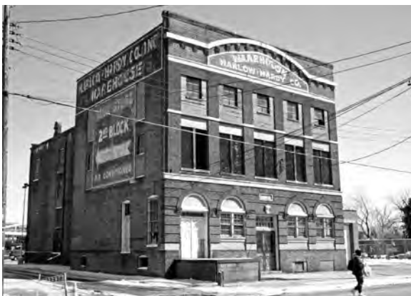
A building in the Atlantic Coast Line Railroad Comm. and Indus. HD
