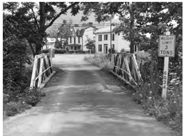
Crab Run Lane Truss Bridge, photo circa 1980
