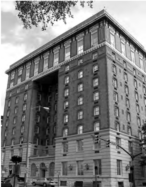
Ninth Street Office Building
