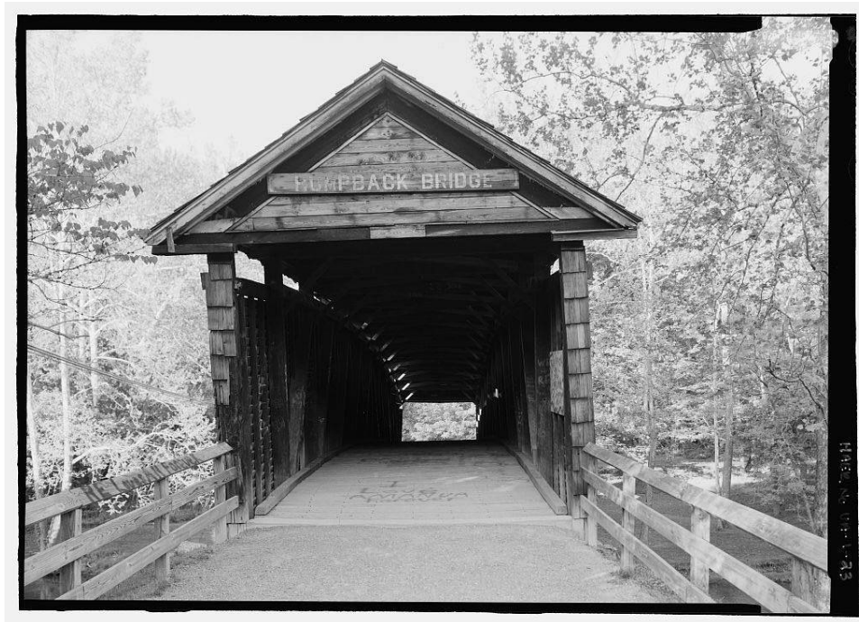
HUMPBACK BRIDGE. West portal elevation. Photograph by Jet Lowe, 2002
