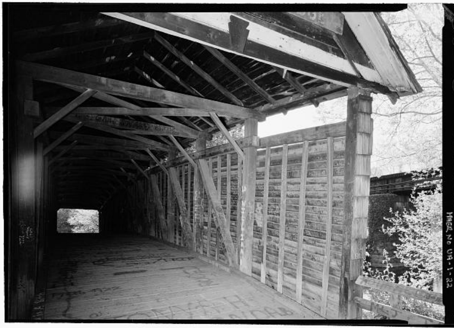
HUMPBACK BRIDGE. Interior view from east portal. Photograph by Jet Lowe, 2002
