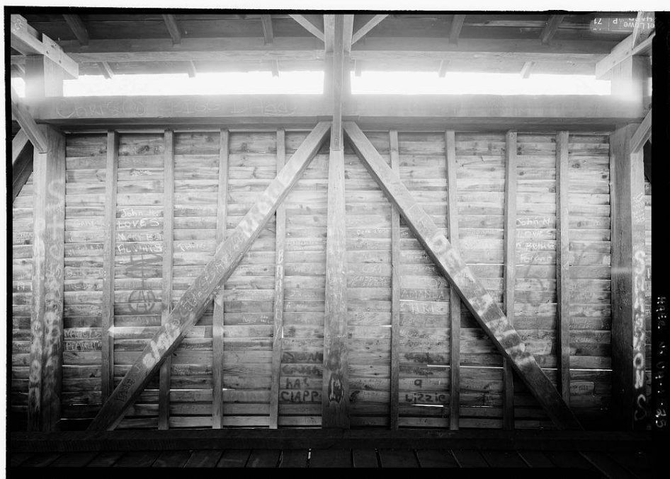
HUMPBACK BRIDGE. Truss detail. Photograph by Jet Lowe, 2002
