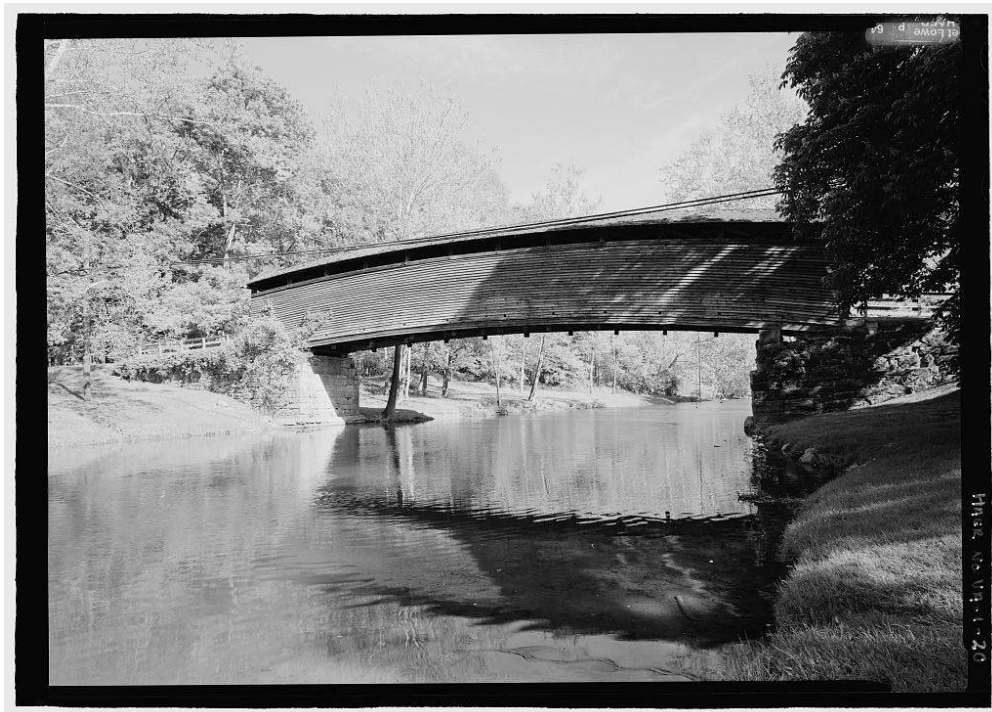
HUMPBACK BRIDGE. Southeast elevation. Photograph by Jet Lowe, 2002
