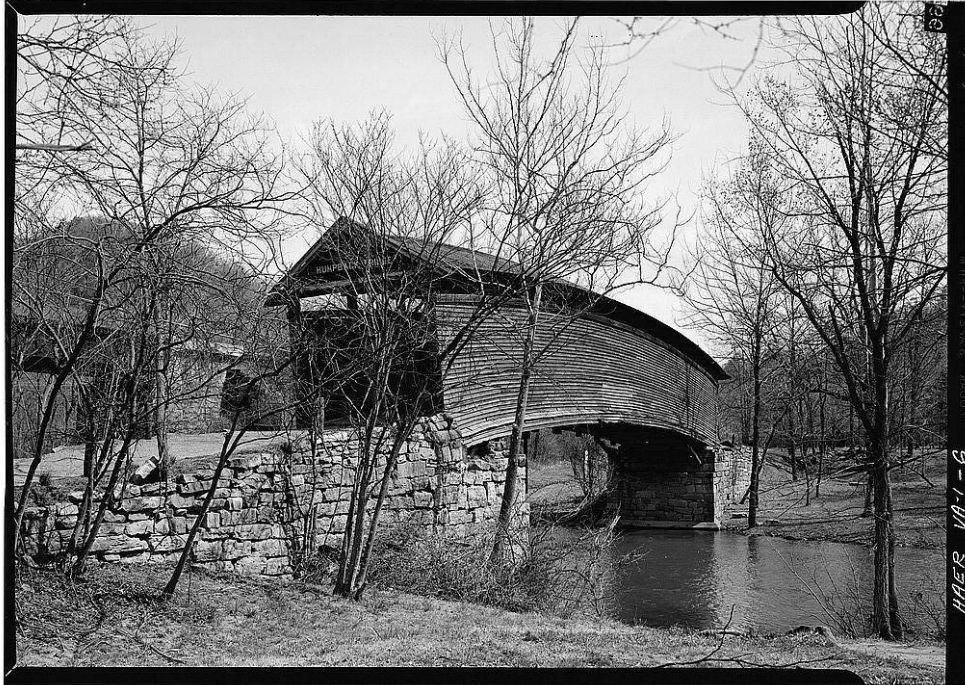
HUMPBACK BRIDGE. General view from southwest. Photograph by Jack Boucher, 1971
