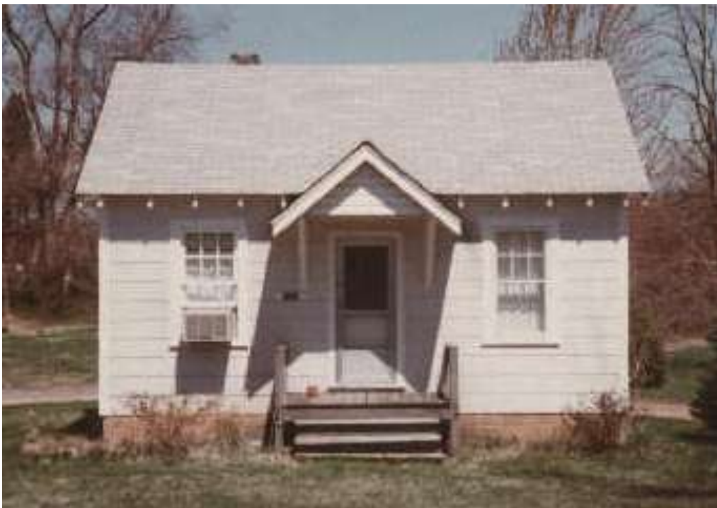
Washington Great Falls & Dranesville Toll House at Leigh Mill Road Rehabilitated as residence. Demolished 2008.
