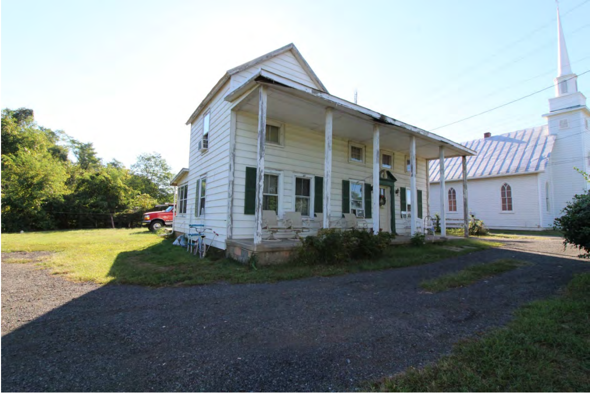
Ca. 1896 Edward Lee House (029-5179-0010; 029-0264) and Floris Methodist Church (029-5179-0009; 029-0263), Looking SE (Maas September 2016)
