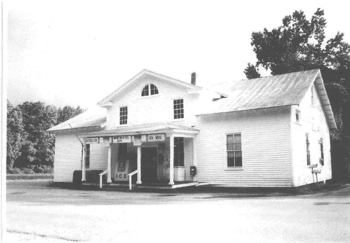
Figure 4. 1990s photograph of the south façade of Ware Neck Store and Post Office.
