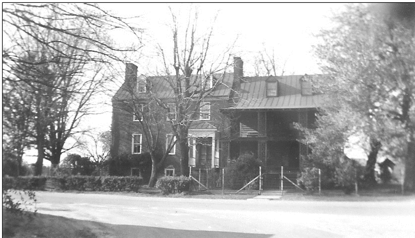
Figure 4. 1947 Photograph of the Tavern at Old Church (Image on file at the Department of Historic Resources, Richmond, VA).
