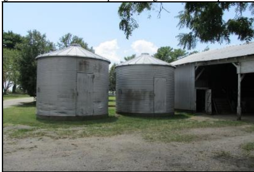
Metal Grain Bins, North Elevation
