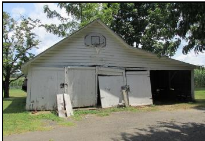
Detached three-car garage, south elevation
