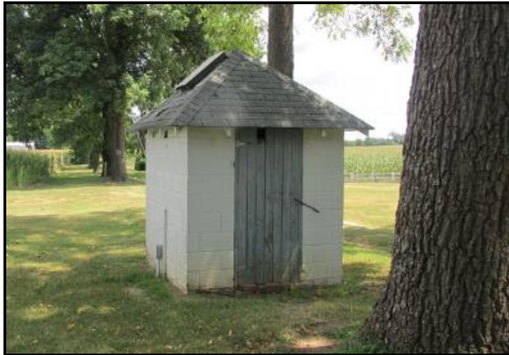
Concrete Block Well House, south elevation
