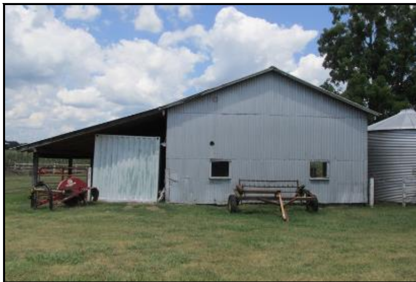
Frame Barn 1, south elevation
