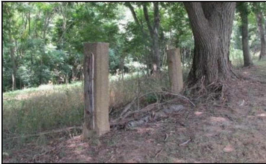
Aggregate Concrete Gate Posts/Piers, View looking southwest
