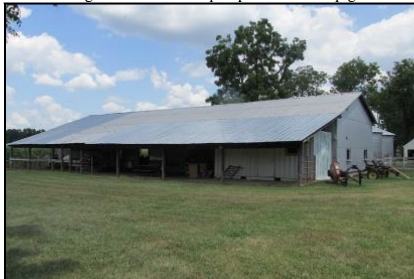
Frame Barn 1, southwest oblique view
