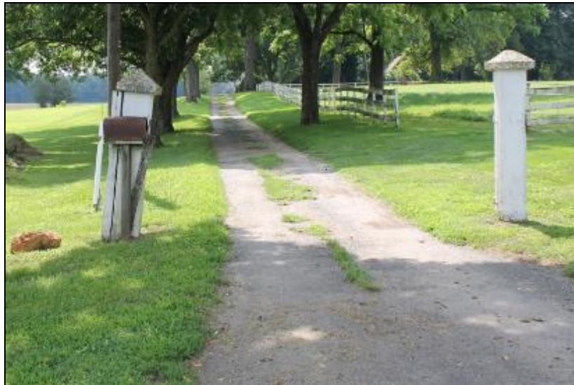
Parged Concrete Posts, View Looking East
