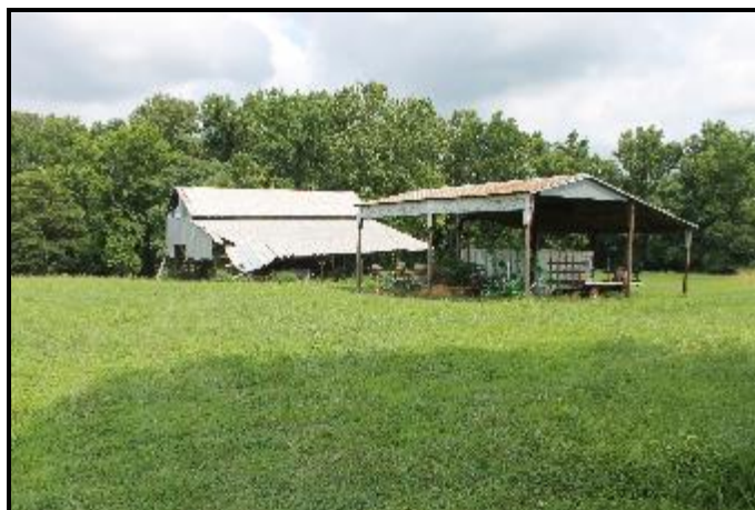
Pole Barn 1 (at right) and Frame Barn 3 (at left)
