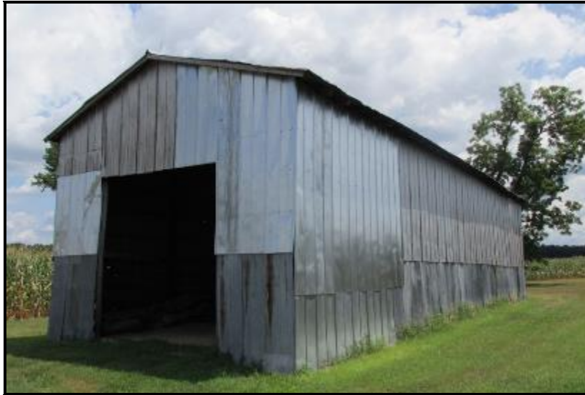
Aluminum Barn, Northeast Oblique View
