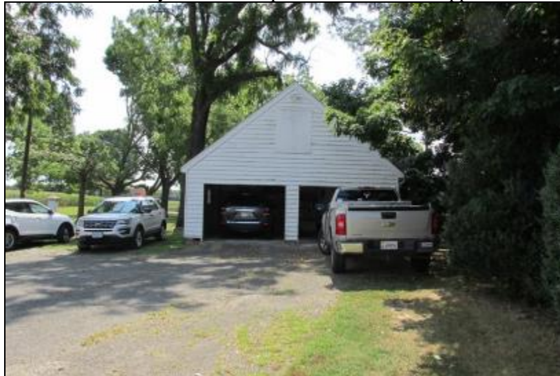
Detached two-car garage, west elevation
