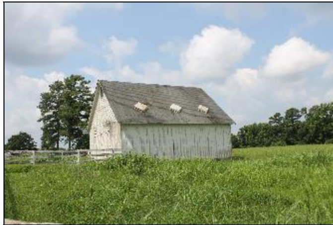
Frame Barn 4, Northeast Oblique View
