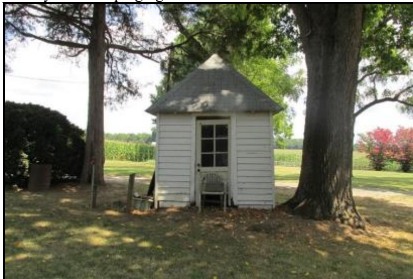
Frame well house, south elevation
