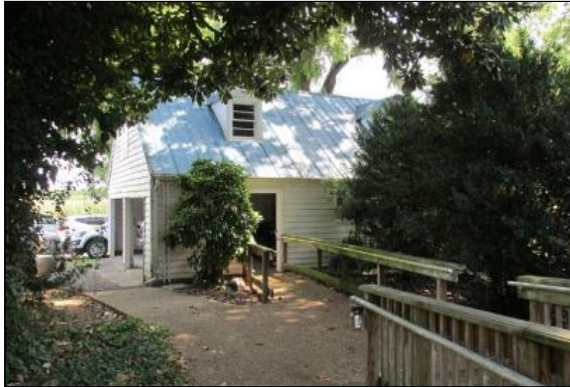
Detached two-car garage, partial view south elevation
