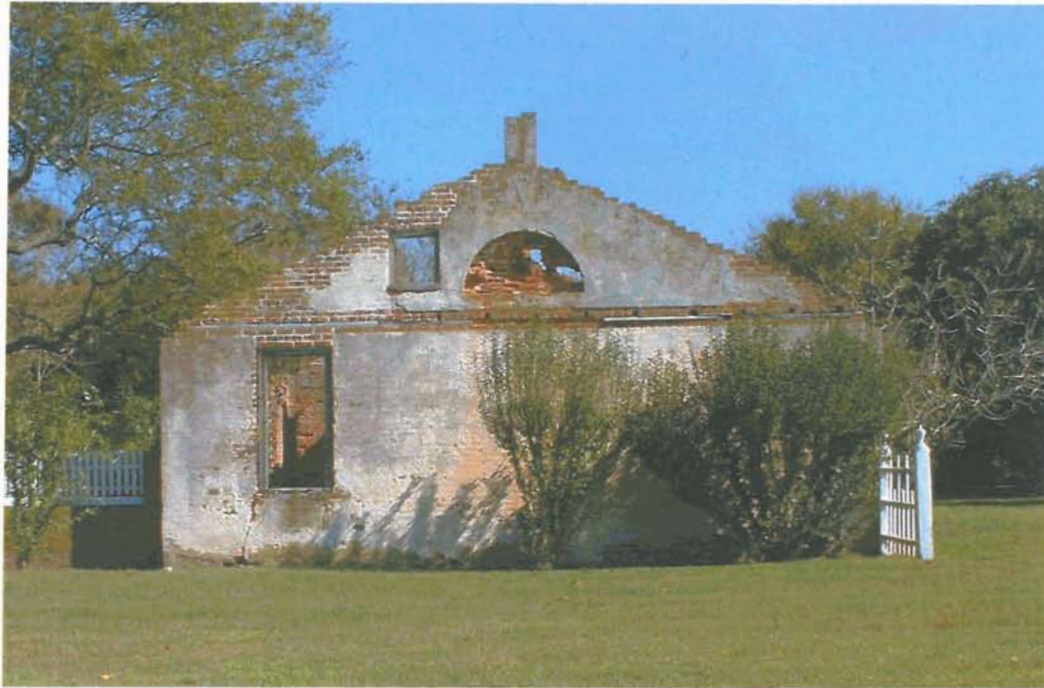
Orangerie, west elevation Michael Bourne, 2004
