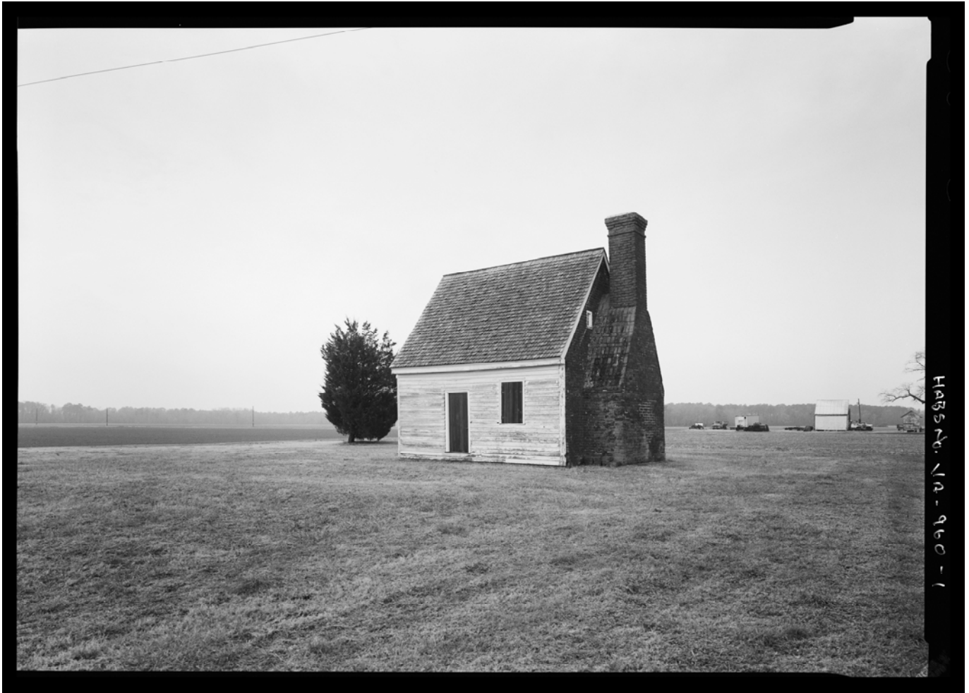
Perspective view looking from the northeast to the east (front) and north gable end Photograph from HABS, James W. Rosenthal, photographer, 2011
