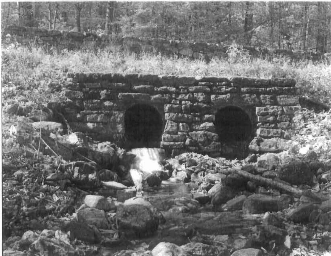
View of Double Culvert. Photograph by William A. Faust II, 1996.
