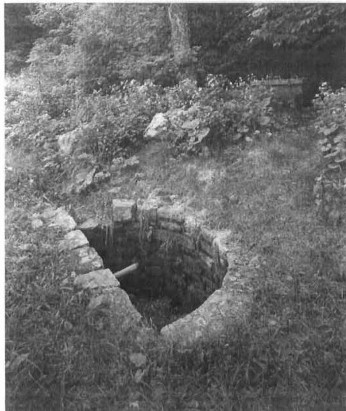
Catch-basin with uphill springhouse. Photograph by William A. Faust II, 1996.
