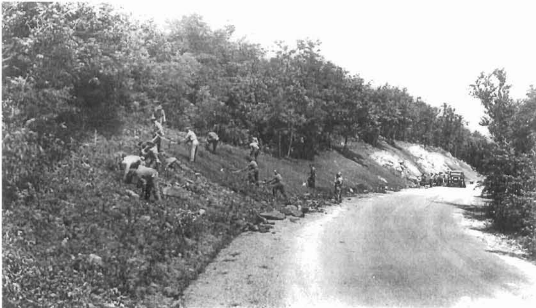
Bank blending by the CCC along Skyline Drive. Photographer unknown, Shenandoah National Park Archives.
