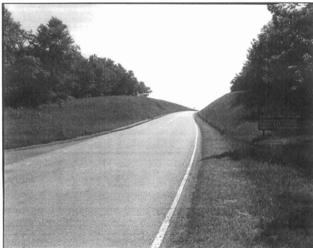
Realigned segment of drive near Big Meadows. Photograph by William A. Faust II, 1996.
