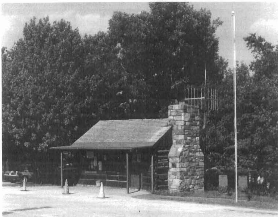
Campground check-in building, Big Meadows. Photograph by William A. Faust II, 1996.
