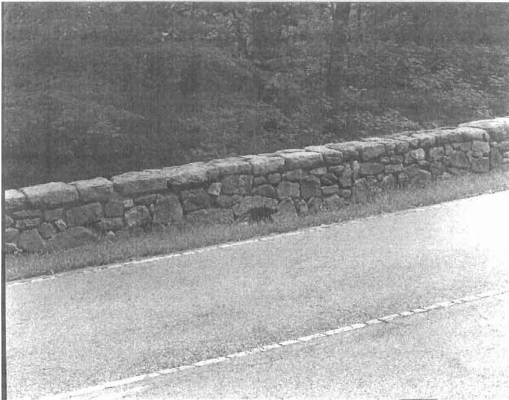
Replacement guardwall, built ca. 1990. Photograph by William A. Faust II, 1996.
