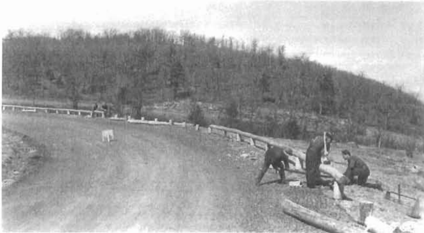
CCC's building log guardrail. Shenandoah National Park Archives (no. P455c)
