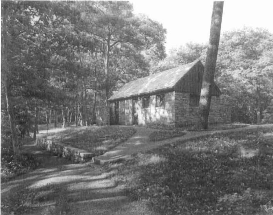
Comfort station at Lewis Mountain, Photograph by William A. Faust II, 1996.
