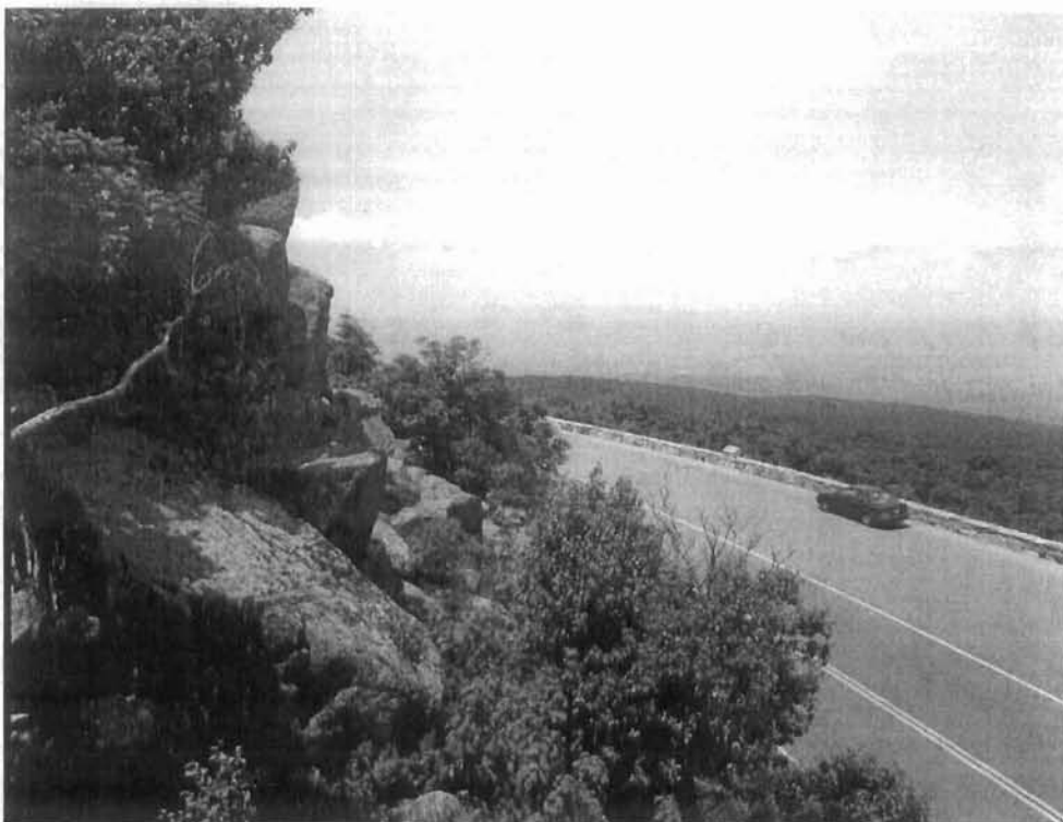
Hogback Overlook looking toward Shenandoah Valley. Photograph by William A. Faust II, 1996.
