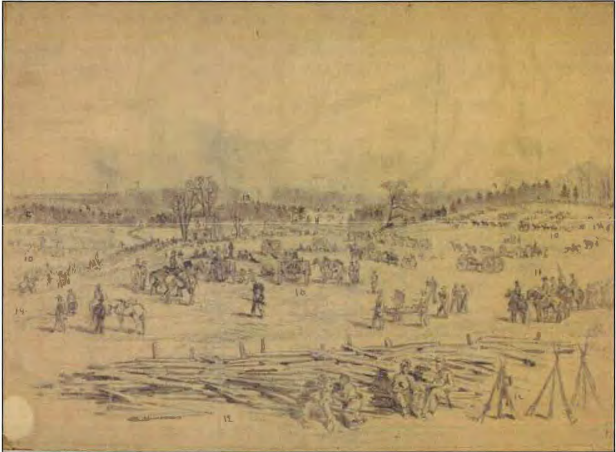
Figure 28. "The battle of Spotsylvania [sic]--View of the field from the center of the position," Edwin Forbes, May 9, 1864 (source: Library of Congress Prints and Photographs Division Washington, DC). Note the reveted breastwork in the foreground, a version of the type of fieldworks that became common features of battlefields as the war progressed.
