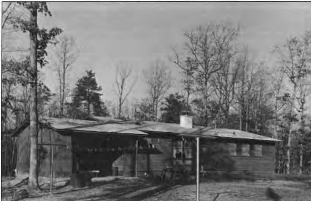
Figure 39. Chancellorsville Ranger Housing, undated (source: National Park Service, Denver Service Center). Photo shows typical housing on Ranger Lane, constructed as part of Mission 66 improvements.
