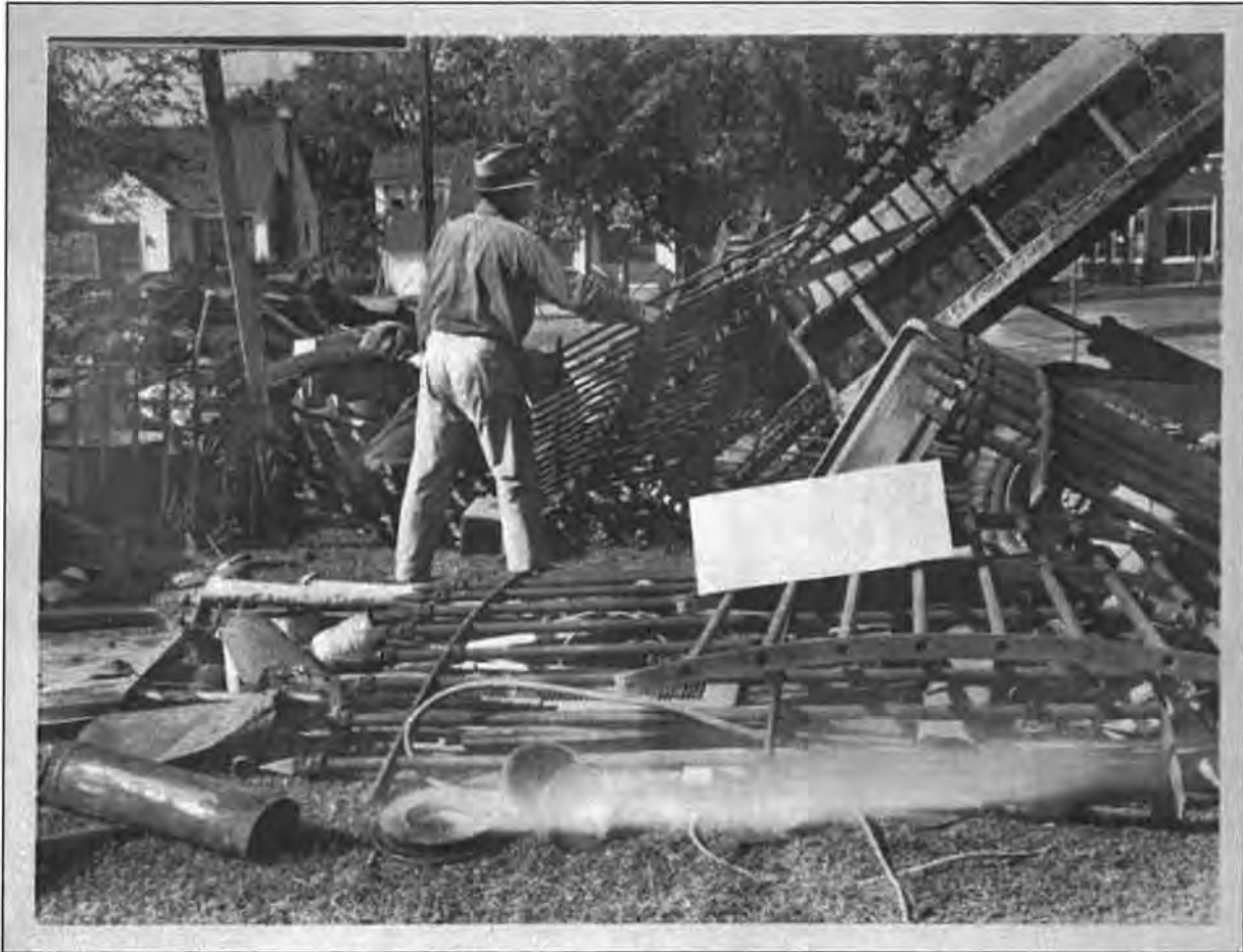
Figure 33. Scrap Metal Drive, Fredericksburg, VA, September 1942 (Image from Central Rappahannock Heritage Center, posted on https://npsfrsp.wordpress.com/2010/07/23/a-patriotic-end-for-some-cool-history-stuff/ ). Photo shows the fence which had surrounded the Jackson monument at Chancellorsville in a pile of scrap metal being collected in support of the World War II effort.
