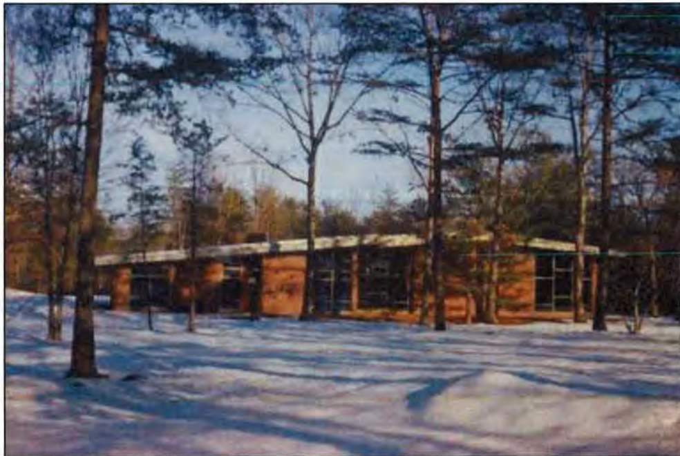
Figure 37. Chancellorsville Visitor Center, 1963 (source: National Park Service, Denver Service Center). Photo shows Chancellorsville Visitor Center, shortly after opening to the public.
