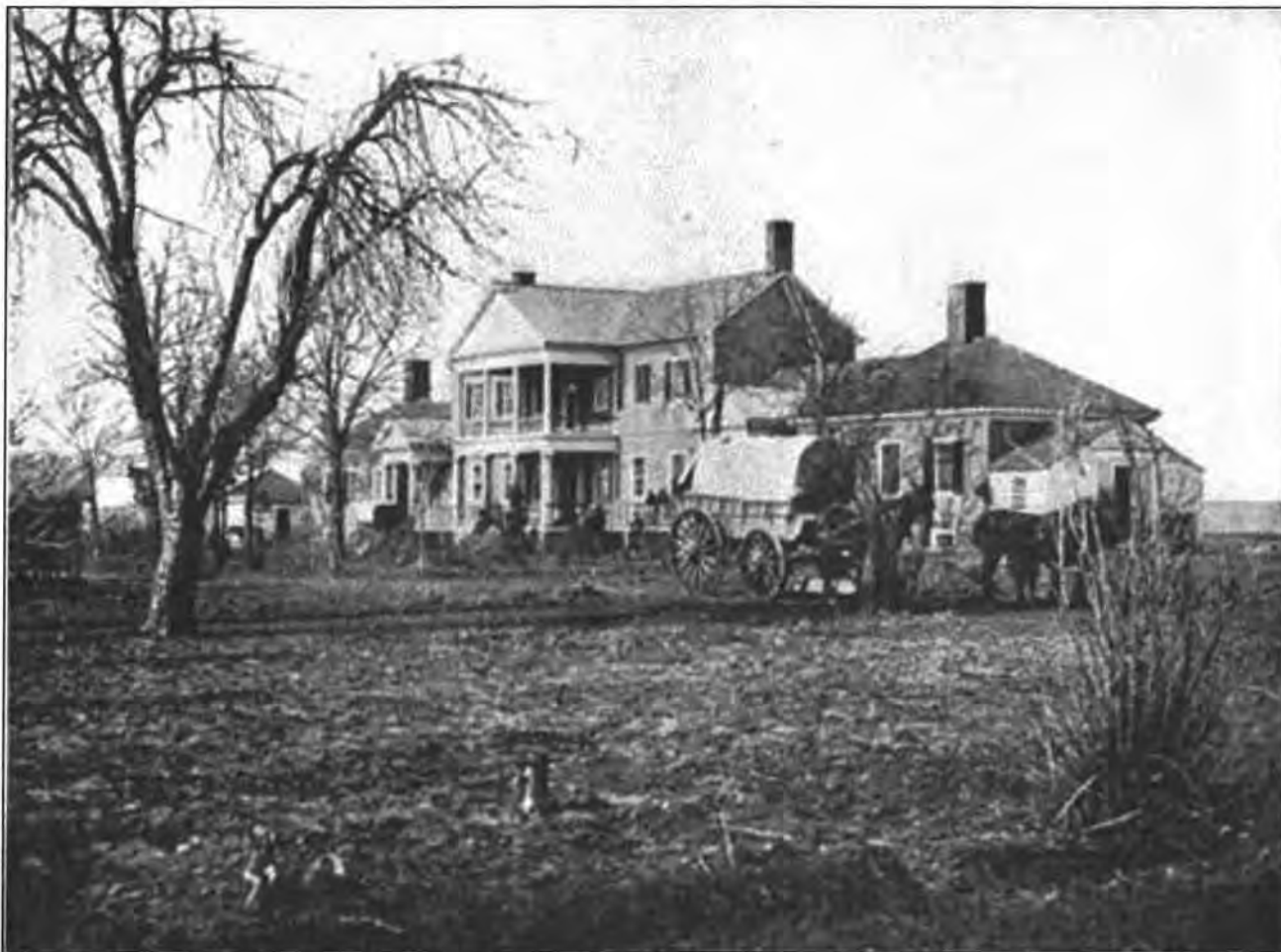
Figure 42. Chatham, ca. 1863 (source: Fredericksburg and Spotsylvania NMP). Photo shows west elevation of Chatham with two-story Greek Revival porch that was removed during ca. 1920 renovations.
