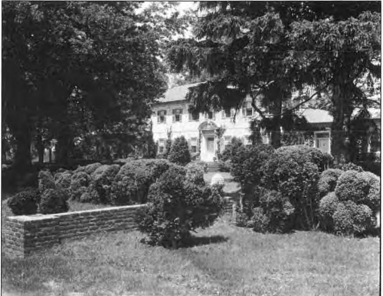
Figure 43. Chatham, Frances Benjamin Johnston, 1929 (source: Library of Congress, Prints and Photographs Division, LC-DIG-ppmsca-16908). Photo shows west elevation of Chatham and west terrace landscape following restoration and landscape work by Oliver Clarke and Ellen Biddle Shipman in the early to mid-1920s. Note the removal of the Greek Revival porch and its replacement with a Classical Revival door surround.
