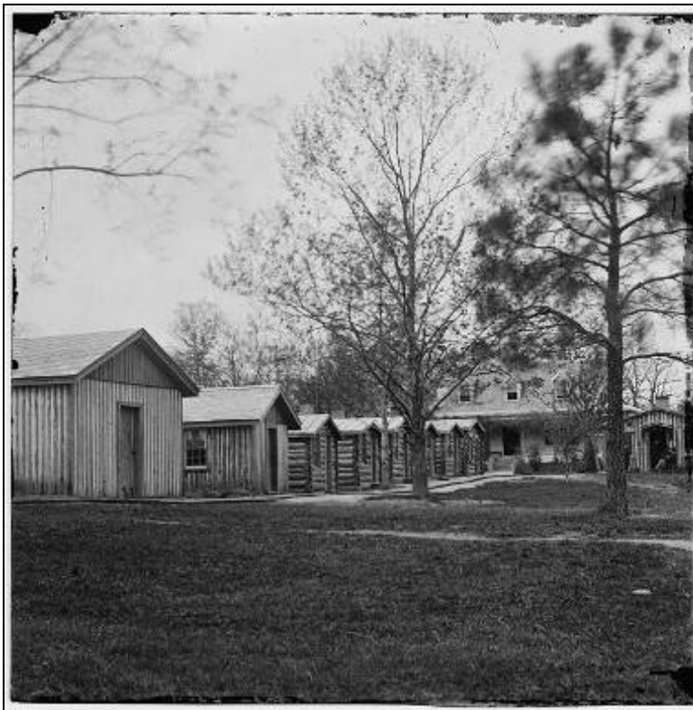
Row of Military Cabins Constructed in front of Appomattox Manor, City Point, Virginia, 1865. Source: Library of Congress, https://www.loc.gov/item/2018671156/ .
