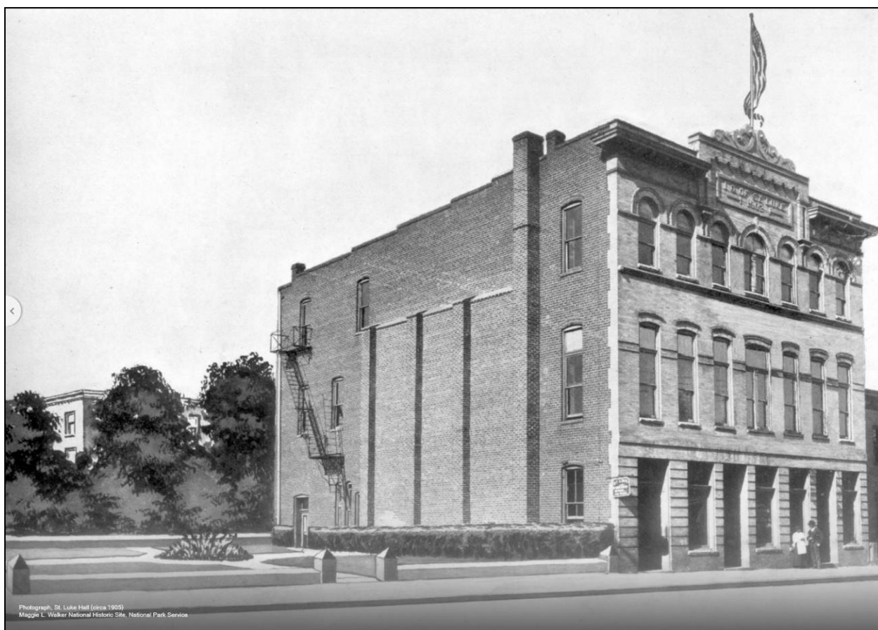
Image 1. The St. Luke Building as it appeared in 1905 (photograph courtesy of Maggie L. Walker National Historic Site, National Park Service, Richmond, VA).
