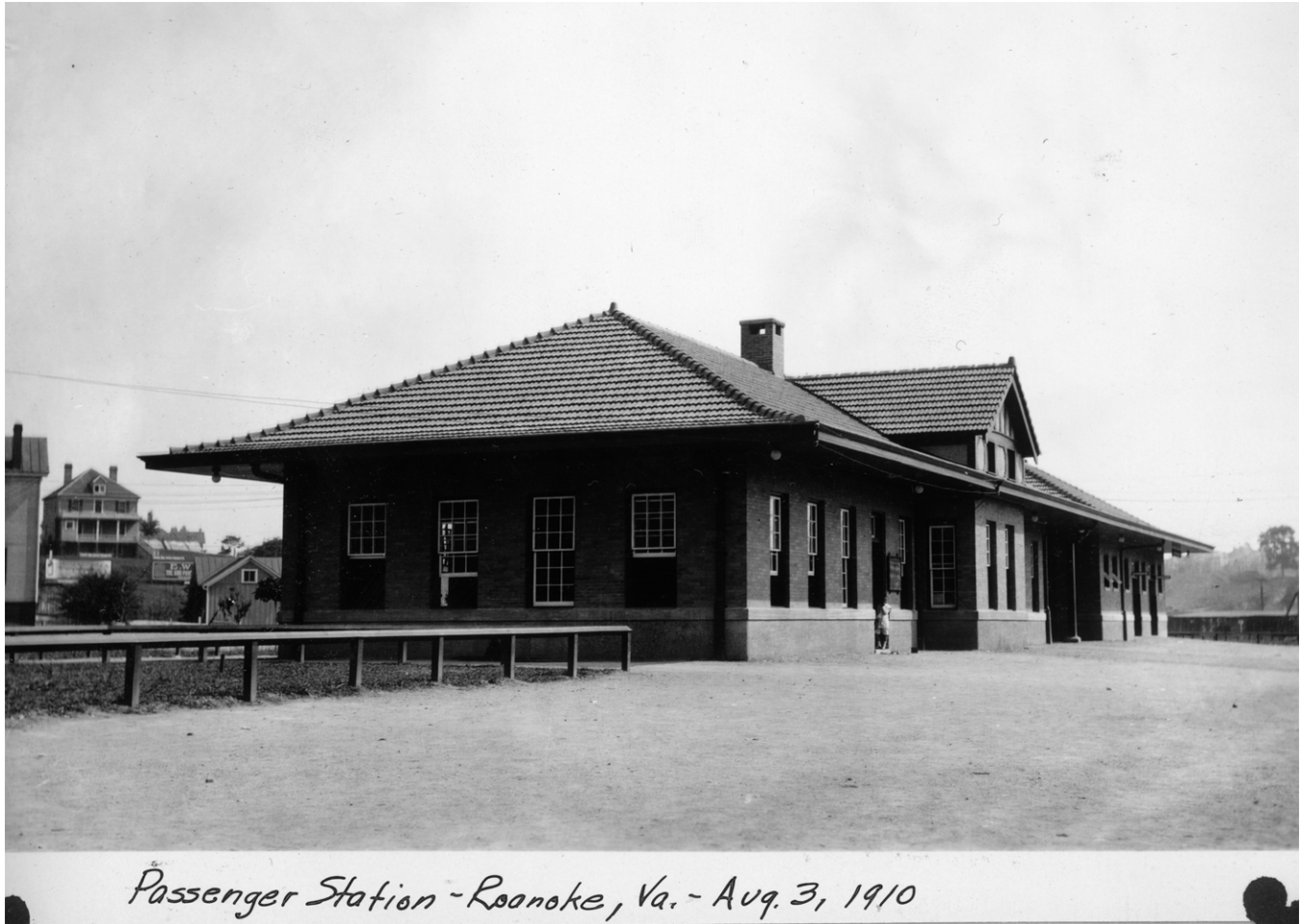
Figure 1: Virginian Railway Passenger Depot, 1910.
