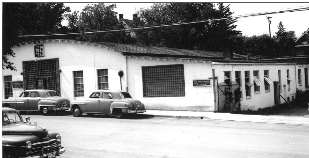
Figure 2.c. 1951 Photograph of the Carpenter Hosiery Mills Building. View west.(Courtesy of the Wythe County Historical Society).
