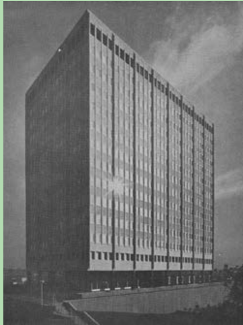
The Madison Building by Hayes, Seay, Mattern & Mattern, Capitol Square, Richmond (Image: from "The James Madison Office Building and Parking Facility," Virginia Record 91.5 (May 1969): 16)
